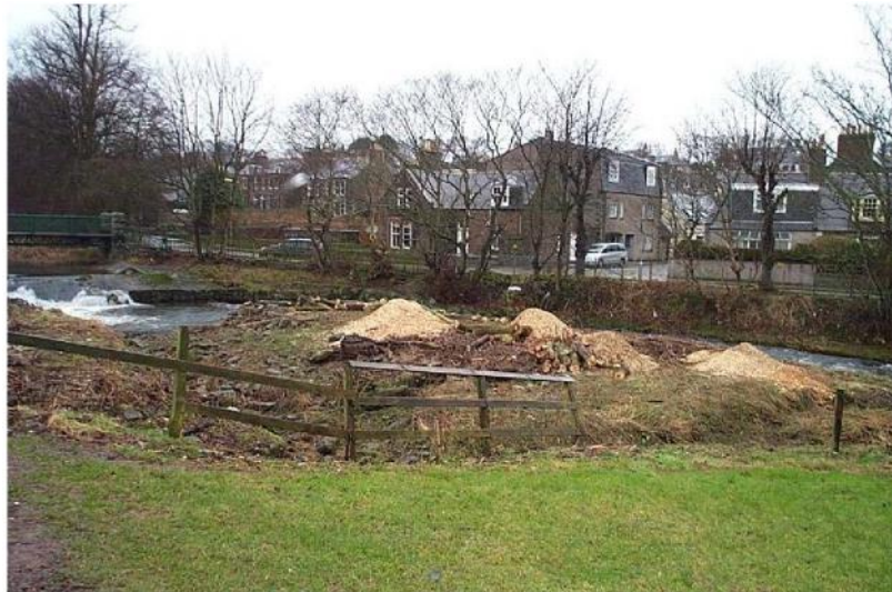
Figure 3 Tree clearing prior to river engineering works
