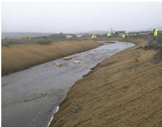
Figure 33 ✓ Good practice: (left) initial installation of biodegradable matting preventing erosion of soil, photo on right shows matting after initial establishment of vegetation
