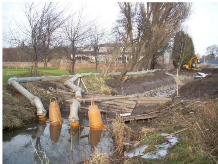
Figure 19 ✓ Good practice: full isolation of channel by over pumping
