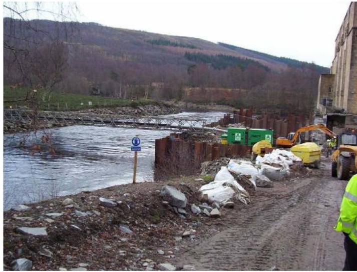
Figure 15 ✓ Good practice: steel piled cofferdam
