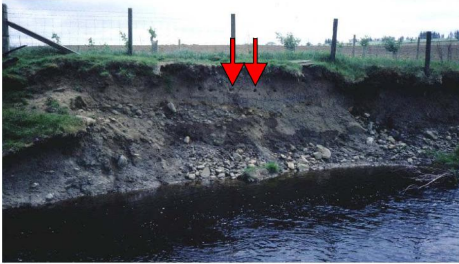
Figure 2 Habitats such as sand martin burrows can be destroyed during the construction phase
