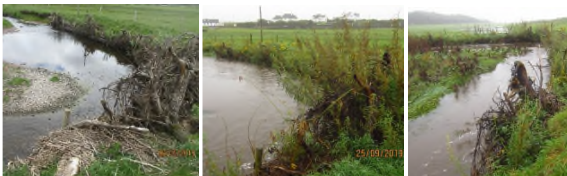
Pictures above showing the works 2 years after completion.
