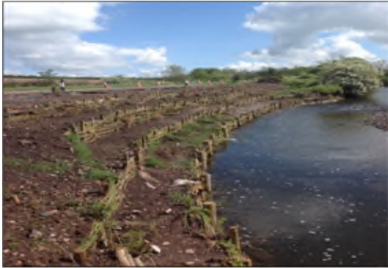
Figure 6a: Examples of recently installed willow spiling for bank protection on a low bank
