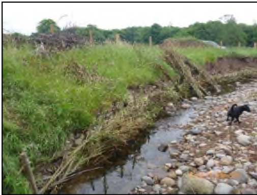
Figure 7: Details of willow stakes and rods installation
