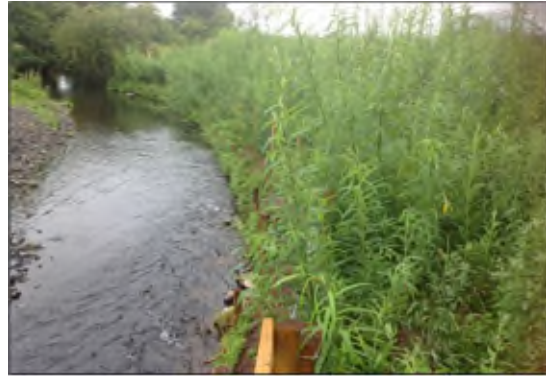
Figure 5b: Terraced willow spiling one year later, viewed from the opposite direction to Figure 5a. Note the complexity and roughness of the bank compared to that in Figure 5a
