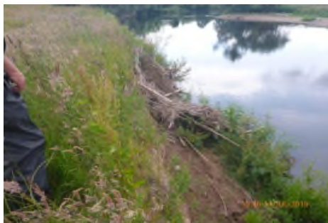
Pictures above showing steep bank with little or no re-profiling, narrow terraces, vertical posts too short and few live stakes all contributing to partial failure.
