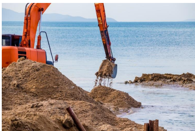
Figure 2- Formation of a pier using land reclamation
