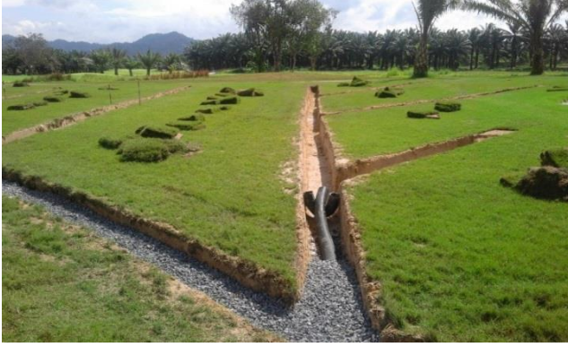
Figure 5- installation of a pipe and gravel drainage system may be an exempt activity
