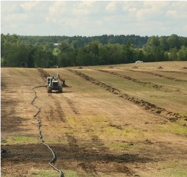
Figure 6- Preparing a rural field for tile draining
