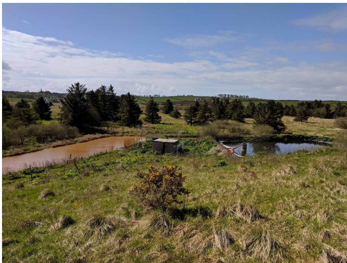
Figure 10 - Leachate lagoons at Tarbolton Landfill site
