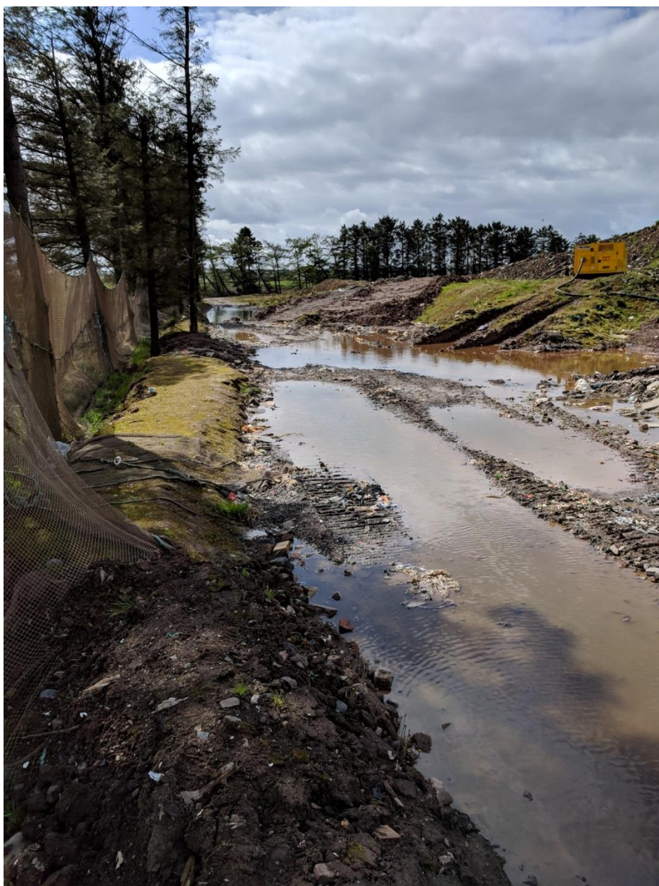
Figure 13 - Water logging of the site track in the east-south east of the site
