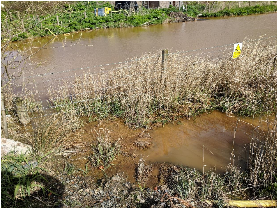
Figure 12 - Flooding of the site path next to the eastern leachate lagoon by overtopped leachate and/or ponded run off
