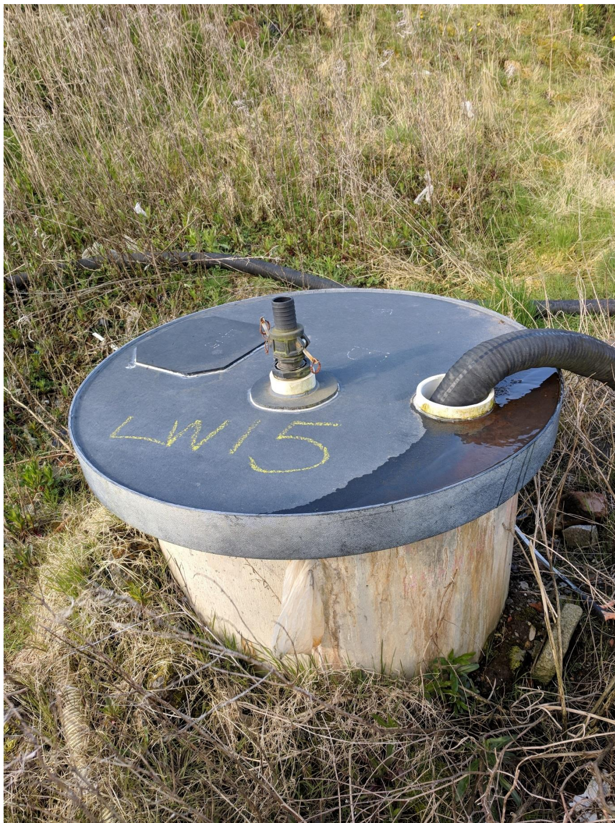
Figure 20 - Chalk marking used on leachate wells which otherwise have no permanent labelling
