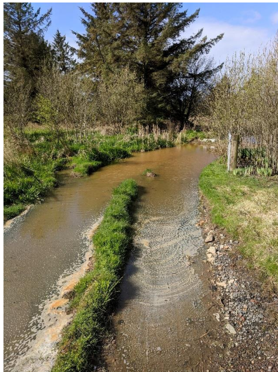
Figure 12 - Flooding of the site path next to the eastern leachate lagoon by overtopped leachate and/or ponded run off
