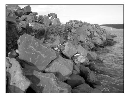
Figure 7.2 Rock armour obscuring a large proportion of the cliff section. Photograph taken looking north east along edge of cliff section.
