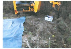
TP3-2-033 Before Excavation 2
