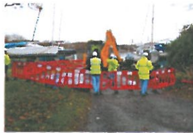
TP3-3-034 Before Excavation (1)
