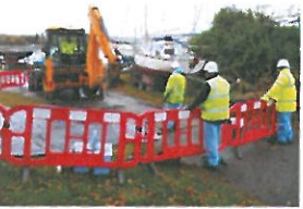
TP3-3-034 Before Excavation (1)
