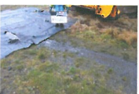
TP3-2-031 Before Excavation
