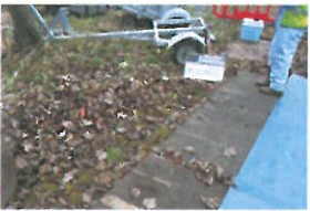
TP3-1-023 Before Excavation
