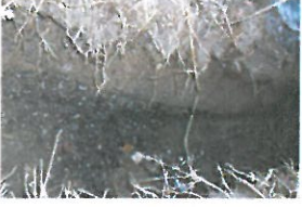
TP3-2-033 Open Excavation (2)
