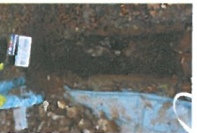
TP3-1-029 Open Excavation 2
