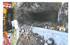
TP3-3-040 Open Excavation
