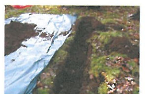
41 Open Excavation at Shallo
