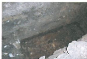
TP3-3-034 Open Excavation (5)
