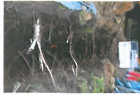
TP3-1-022 Open Excavation
