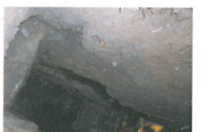
TP3-1-026 Open Excavation 4 (37)
