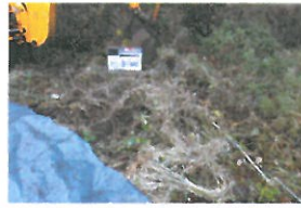
TP3-2-033 Before Excavation 1
