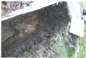
TP3-1-028 Open Excavation 3
