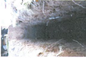
TP3-1-027 Open Excavation
