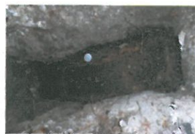
P3-3-040 Open Excavation (3
