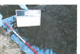
TP3-3-046 Open Excavation (3) 1
