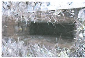
TP3-1-025 Open Excavation 6 (21)
