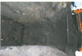
TP3-3-034 Open Excavation (4)
