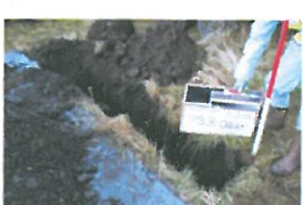
TP3-3-046 Open Excavation (5) 2
