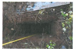
TP3-1-025 Open Excavation (22)
