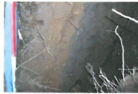
TP3-1-024 Open Excavation (11)
