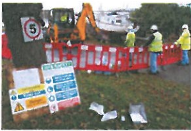
TP3-3-034 Before Excavation (1)
