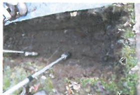
TP3-1-028 Open Excavation
