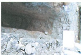
TP3-3-036 Open Excavation (5)
