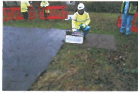
TP3-3-035 Before Excavation (1)
