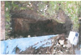
TP3-1-028 Open Excavation 2
