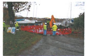
TP3-3-034 Before Excavation (1)
