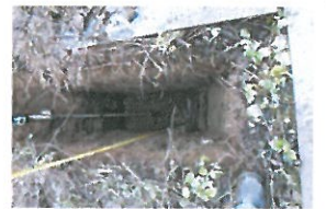
TP3-1-025 Open Excavation 2 (17)
