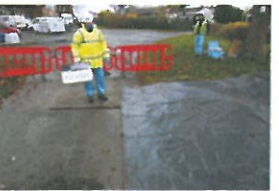
TP3-3-034 Before Excavation (1)
