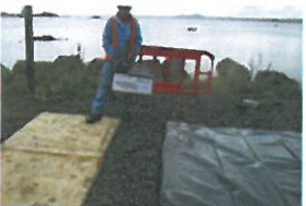
TP3-3-036 Before Excavation (2)
