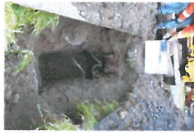
P3-3-039 Open Excavation (2
