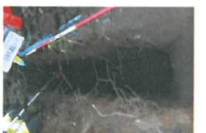
P3-1-024 Open Excavation (8)
