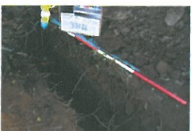
P3-1-024 Open Excavation (7)
