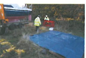
TP3-3-046 Before Excavation (2) 2
