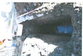
TP3-3-037 Open Excavation
