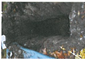
P3-3-040 Open Excavation (2
