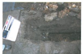
TP3-3-034 Open Excavation (6)
