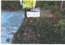
TP3-1-025 Before Excavation (14)
