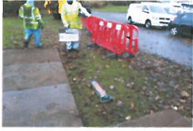
TP3-1-022 before Excavation 2
