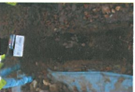
TP3-1-029 Open Excavation
