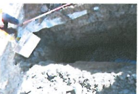
TP3-3-037 Open Excavation (3)
