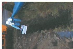
TP3-3-045 Open Excavation 3
