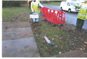
TP3-1-022 Before Excavation
