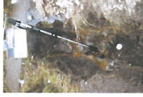
P6-2-061 Open Excavation (16)
