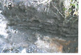
P6-2-063 Open Excavation (20)
