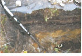
P6-2-061 Open Excavation (14)
