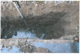
TP6-2-064 Open Excavation (5)
