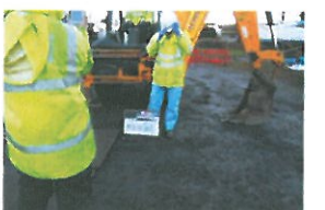
TP3-3-106 Before Excavation (2)
