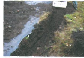
P6-2-061 Open Excavation (10)
