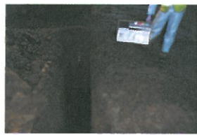
TP3-3-106 Open Excavation 2
