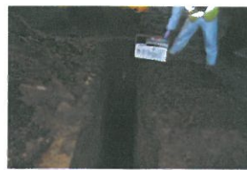
TP3-3-106 Open Excavation
