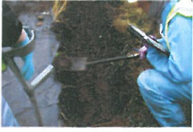
P6-2-061 Open Excavation (7)
