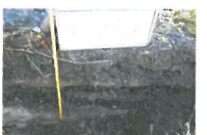
P6-2-053 Open Excavation (3)
