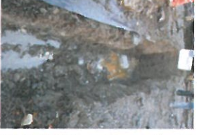
P6-2-062 Open Excavation (4)
