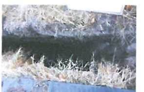
P6-2-060 Open Excavation (3)
