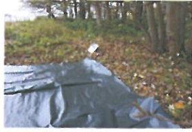
P6-2-063 Before Excavation and Sealing
