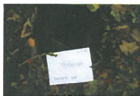
P5-2-049 Open Excavation (5)
