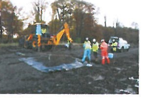
P6-2-062 Spoil and Excavation Area
