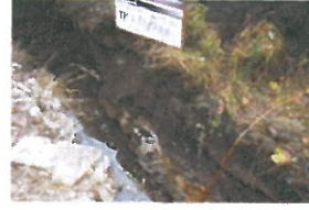
P6-2-061 Open Excavation (17)
