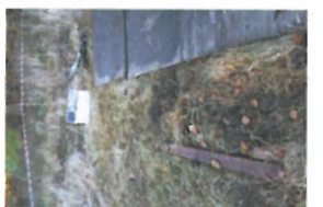
P6-2-060 Before Excavation (2)
