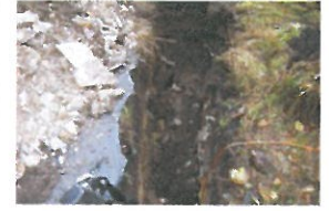
P6-2-061 Open Excavation (18)
