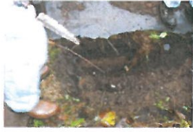
P6-2-061 Open Excavation (8)
