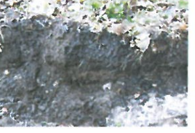
P6-2-063 Open Excavation (4)
