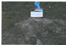
TP6-2-054 Restored Surface (2)
