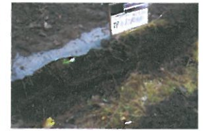
P6-2-061 Open Excavation (11)
