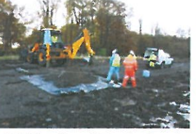
P6-2-062 Spoil and Excavation Area
