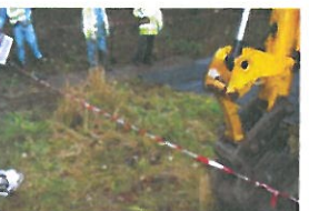
P6-2-061 Before Excavation (2)
