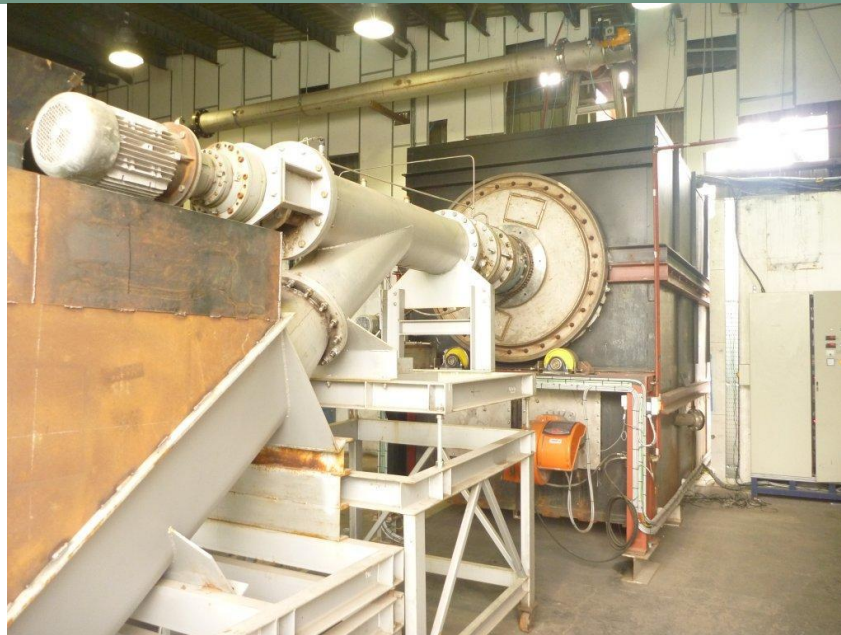
Photo 3: Drum Pyrolysis Chambers
