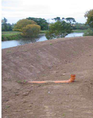
Figure 8. Outlet pipe with an adjustable bend.
