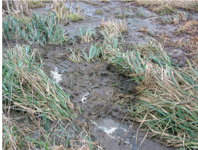
Figure 15: Sediment accumulation in the initial cell of a CFW.
