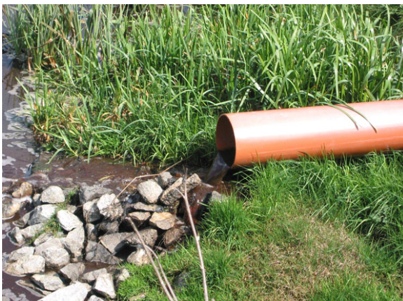
Figure 7: Inlet pipe to CFW cell
