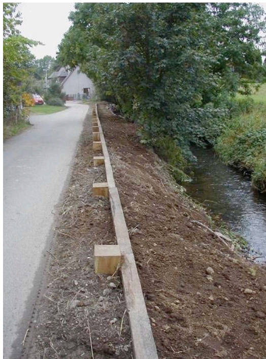
Figure 2 ✖ Poor practice: bare soil as a result of flood prevention works (photo courtesy of Kathy Dale, NES)
