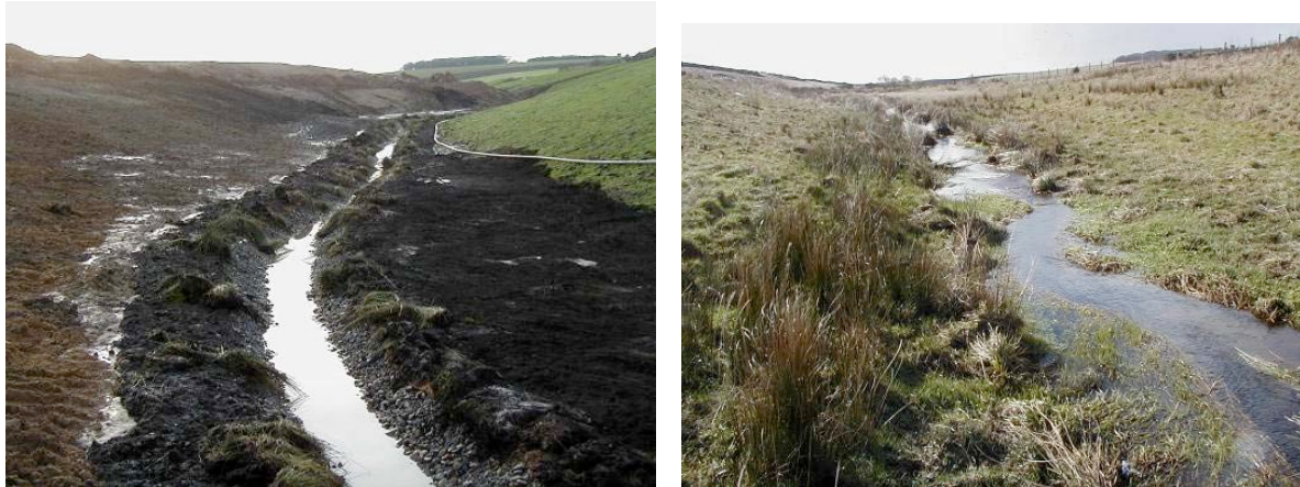
Figure 3 ✓ Good practice: transplanting of soft rush during construction and two years later (photos courtesy of Kathy Dale, NES)
