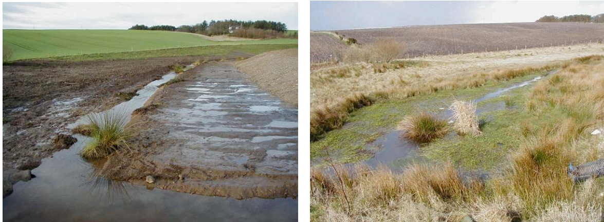
Figure 11 ✓ Good practice: berm creation on the right of the channel and the berm two years later
