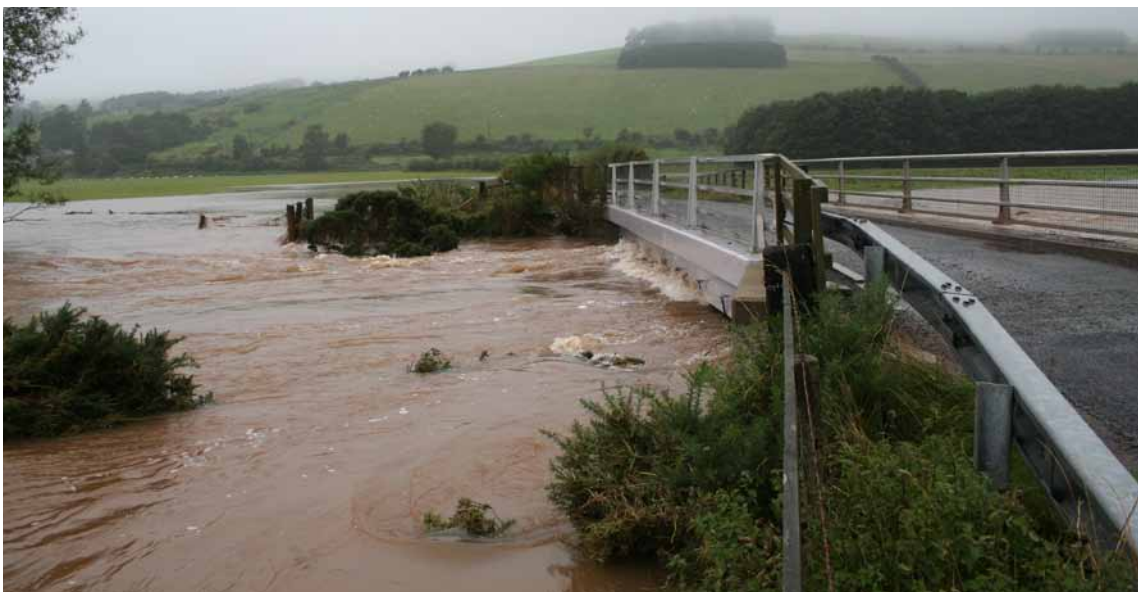
Figure 16: Crossings can constrict flood flows which can increase bank and bed erosion and alter sediment deposition, damaging river habitats and crossing structures.
