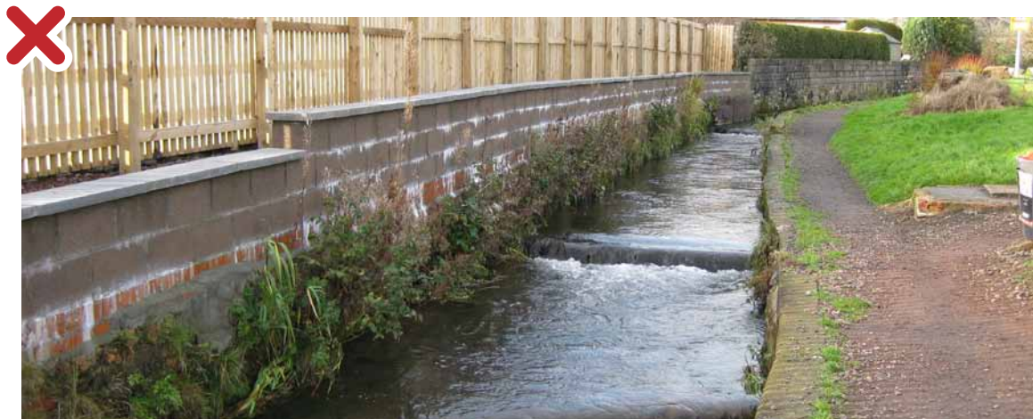
Figure 55: Poor practice, pipeline laid in the river channel. Can cause scour around the structure and pipe is at risk of damage during high flows.
