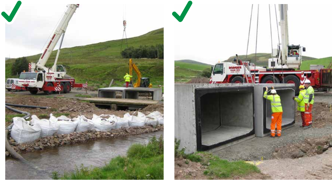
Figure 56: Good practice, works area has been isolated and kept dry by a temporary diversion (left) to allow installation of a culvert (right) that requires working in the river bed.
