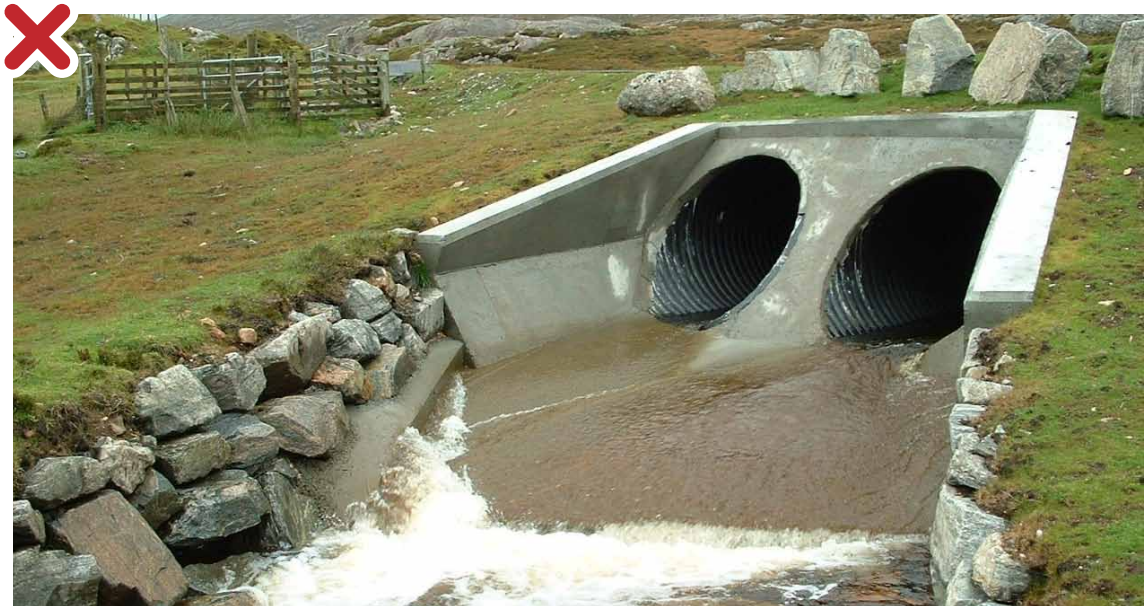
Figure 4: Poor practice. A bridge invert may be level with the riverbed at the time of construction but subsequent erosion downstream due to scour can lead to a drop forming (perched invert) that can create a barrier to fish passage, it can also lead to flows that are too shallow for fish to swim through.
