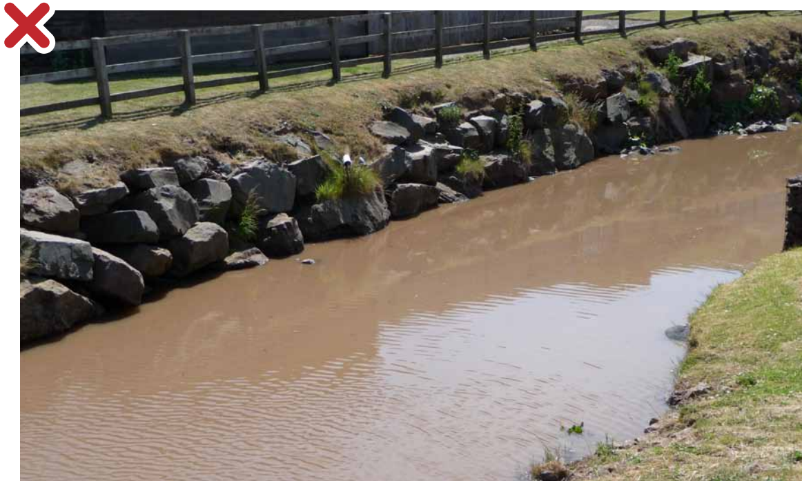
Figure 2: Poor practice. Release of fine sediments during the construction phase can pollute watercourses leading to loss of, or damage to, protected species and habitats such as fish spawning areas.
