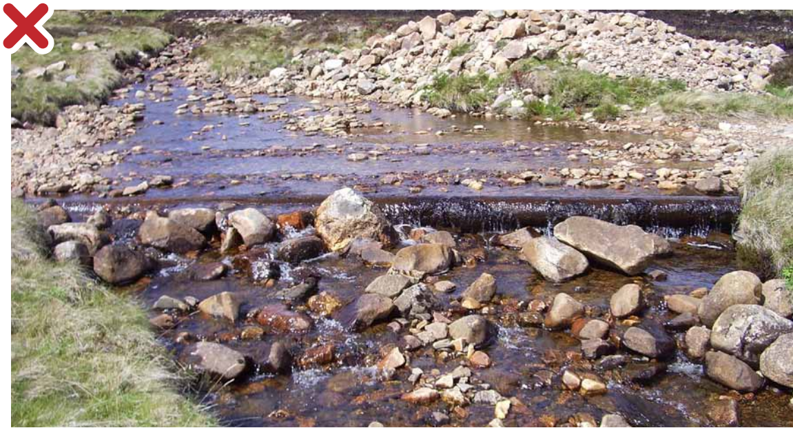
Figure 7: Poor practice. This ford has widened the river, leading to flows that are too shallow for fish to swim through. Photograph courtesy of the River Dee Trust.
