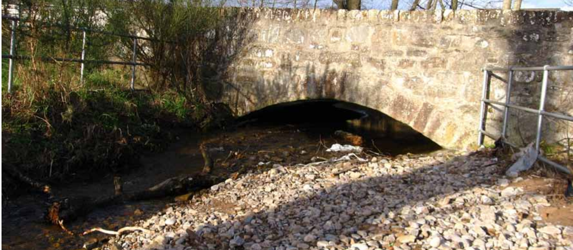
Figure 10: Increased sediment deposition at a bridge can increase flood risk
