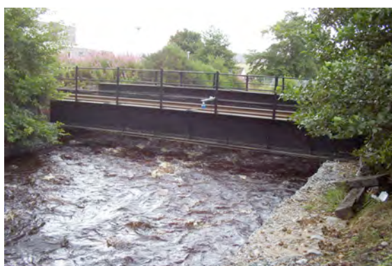
Figure 31: Sediment can accumulate at crossings which may lead to a risk of flooding.
