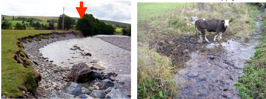
Figure 18 Left: This picture shows no erosion and stable banks where trees are present (see where arrow points) but significant erosion where bank-side vegetation has been removed, resulting in the banks being weakened. Right: Weakened bank due to lack of vegetation and 'poaching' from livestock.
