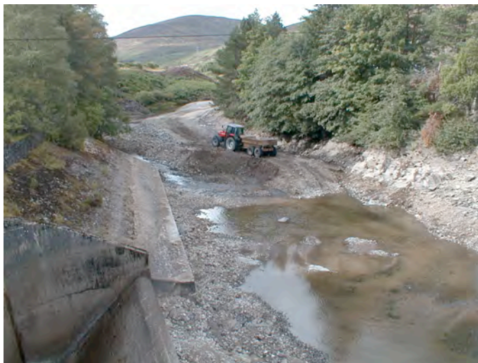
Figure 33: Sediment removal from behind an impoundment. Photograph courtesy of Scottish and Southern Energy.
