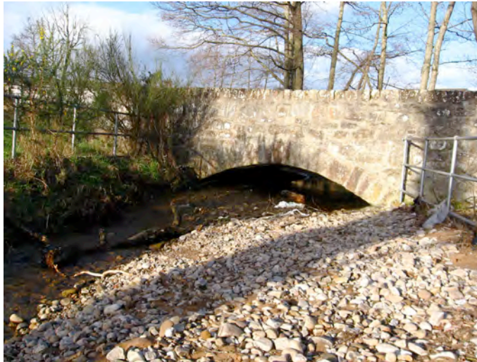
Figure 23: Sediment deposition at a bridge can increase flood risk.
