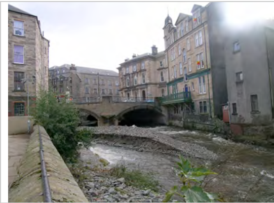
Figure 29: Gravels in the River Slitrig at Hawick. Modelling showed that removing gravel did not have a significant effect on water levels during the one in 200 year event.
