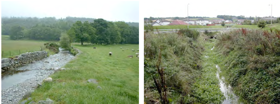
Figure 22: ✘ Inappropriate design in modified channels: both rivers have less energy and are unable to transport sediment, leading to increased deposition. In the left photo, the river bed level is now above the flood plain.
