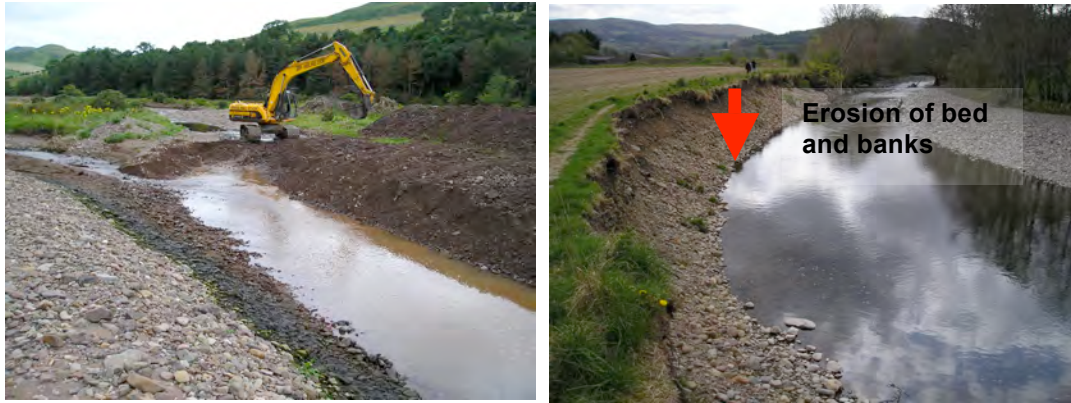
Figure 21: X Left: inappropriate channel design and removal of armour layer leading to the river having more energy, and increased rates of erosion. Right: increased erosion of bed (bed has incised) and banks after a 'knick point' created significant instability.
