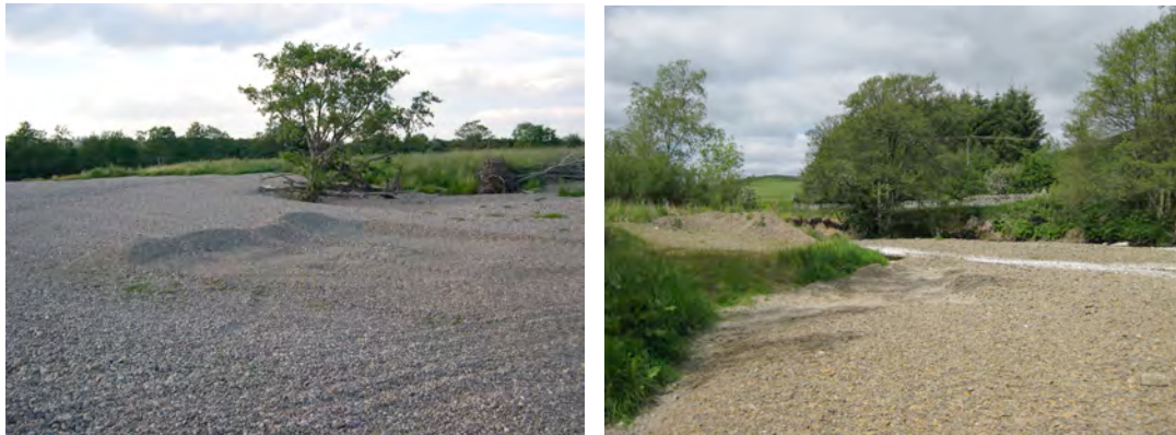
Figure 34: ✓ Good practice: small areas of sediment removed from dry deposits with no holes or pits formed (sediment is 'skimmed' from the top of the dry deposits).
