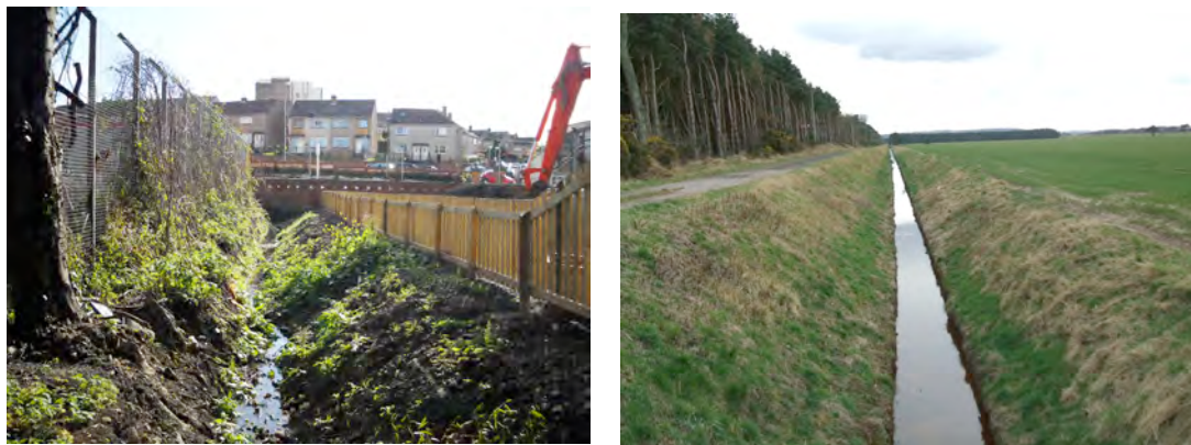
Figure 40: Burns that have been artificially straightened and dredged in the past.
