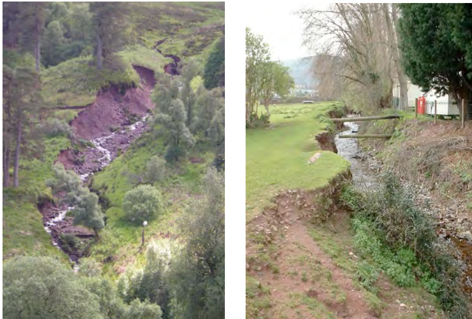
Figure A5: Incising river reaches. Note very extensive erosion of banks and obviously lowered bed.
