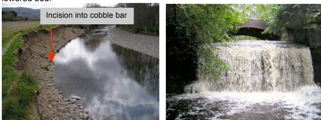
Figure A6: Incising river reaches. Left, note the bed has incised vertically about 2m through the cobble bar (note the vertical bar face and exposed roots). Right, note vertical drop of approximately 4m downstream of a bridge, weir and bank reinforcement required to prevent bridge from being undermined and collapsing.
