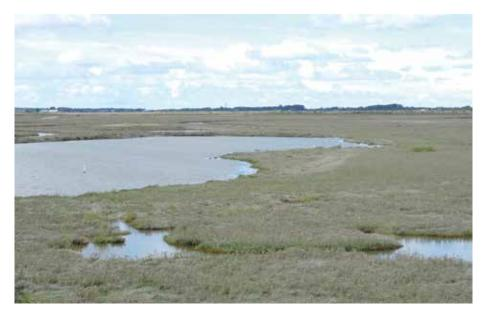
Figure 3.9. Managed realignment and saltmarsh restoration at Hesketh Out Marsh, Ribble Valley Lancashire: Breaches were made in existing defences to create a new line of setback defence and encourage saltmarsh regeneration.
