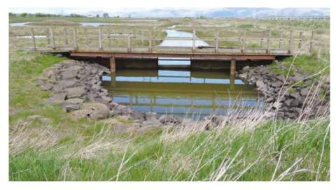
Figure 3.11. Regulated tidal exchange at Skinflats, Firth of Forth estuary: a pipe and sluice (pictured) mechanism was installed to regulate the inflow of sea water onto a grass field, providing a new line of defence and creating new habitat.
