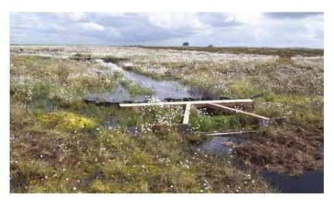
Figure 2.17. Restoration of blanket bog by blocking wide drains using plastic piling supported by timber frames at Blawhorn Moss, West Lothian.
