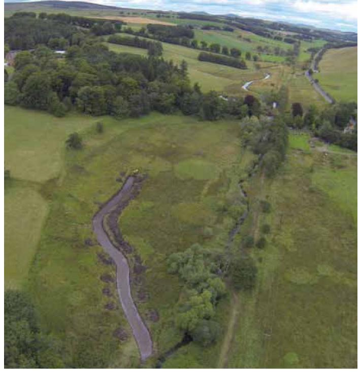
Figure 6.1. Remendering works taking place on the Eddleston Water, Scottish Borders (© Tweed Forum).
