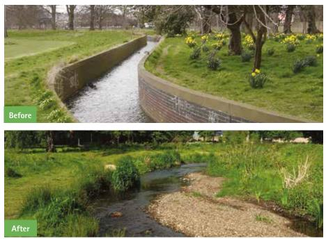
Figure 2.27. The Braid Burn, Edinburgh, before and one year after work to lower an artificial raised bank and replace the concrete channel with sinuous meanders: This work formed part of wider flood alleviation works carried out by the City of Edinburgh Council that sought to also improve biodiversity and public amenity on this watercourse (© River Restoration Centre).
