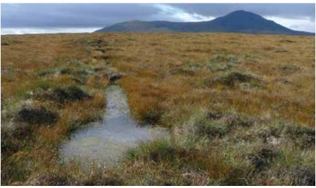
Figure 2.16. Restoration of blanket bog by blocking small drains using peat dams at Forsinard Flows Nature Reserve, Caithness and Sutherland.
