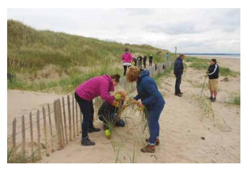
Figure 3.17. Sand dune restoration at St Andrews West Sands, Fife: Beach recharge, sand dune reprofiling and restoration was undertaken to improve the resilience of the dunes to manage flood and erosion risk (© R. Strachan/Fife Coast and Countryside Trust).
