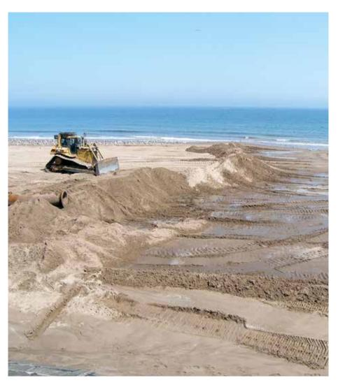
Figure 3.20. Recharge underway at Aberdeen beach to protect sea defences and dissipate wave energy.
