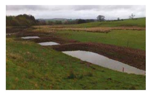
Figure 2.21. Three sediment traps constructed in series to intercept surface runoff and encourage settling out of sediment in the River Coquet catchment, Northumberland (<sup>©</sup> Nick Barber, Newcastle University).
