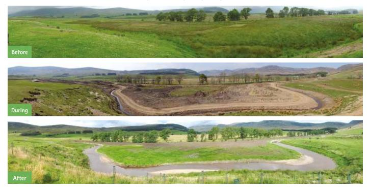
Figure 2.26. The Rottal Burn (South Esk), Angus, before, during and after work led by the Esks Rivers and Fisheries Trust to reintroduce meanders to a channelised reach: In addition to reducing flood peaks, this work sought to improve riparian and aquatic habitat and reduce the unnaturally high sediment load experienced downstream of the reach.
