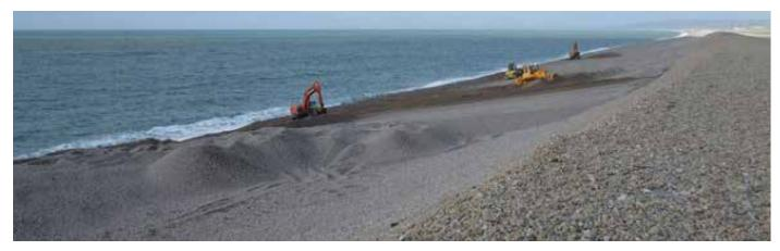
Figure 3.18. Replenishment and reprofiling on the shingle at Chesil beach, Dorset: This work was undertaken in order to increase protection to the community of Chiswell following significant storms (<sup>©</sup> Environment Agency).
