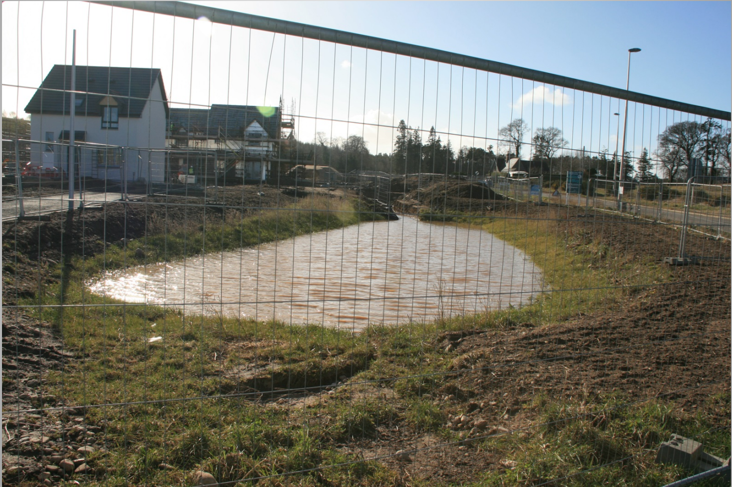
Construction phase SuDs scheme
