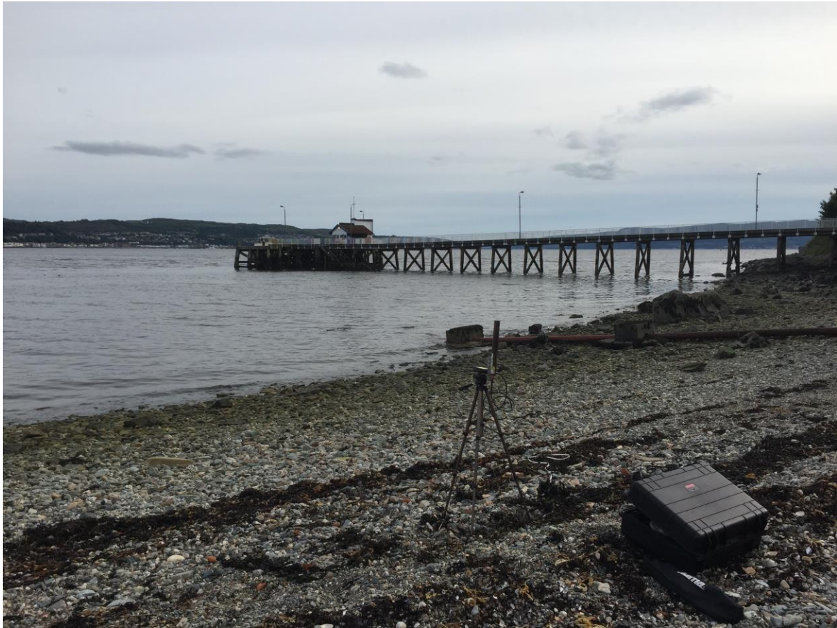
Figure A8i View looking South at Kilcreggan Pier and across the Clyde to Gourrock (July 2016).
