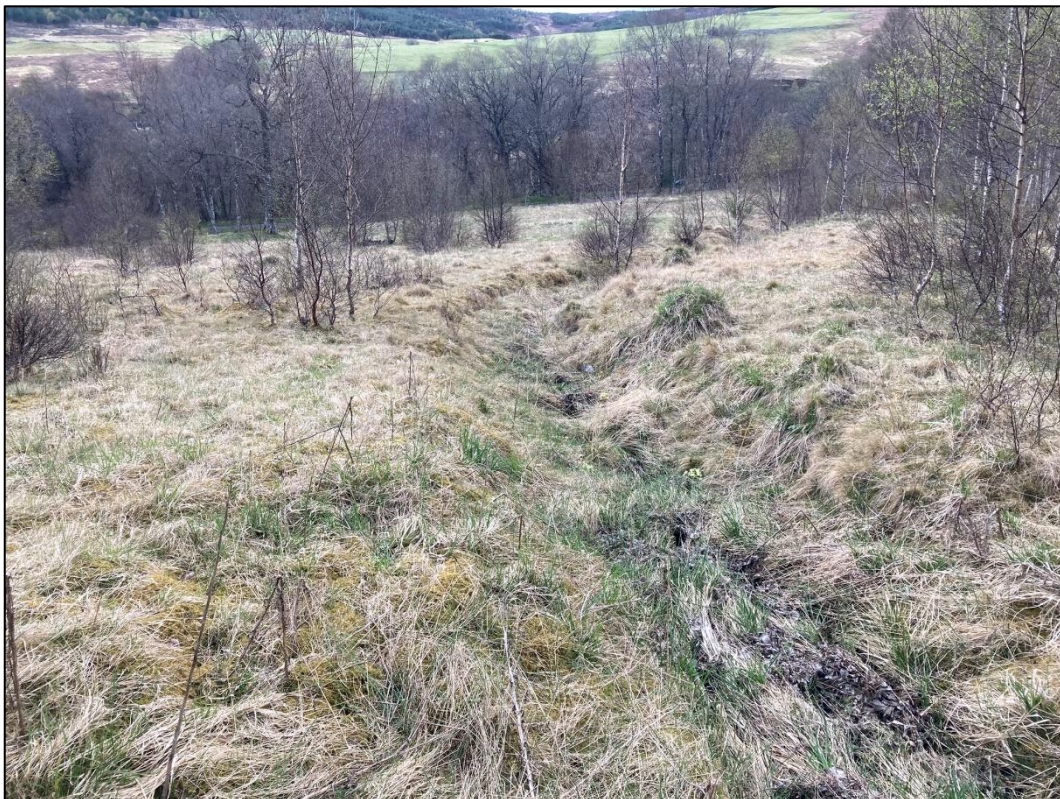
Example of a channel dug to convey roadside drainage downstream of an A road
