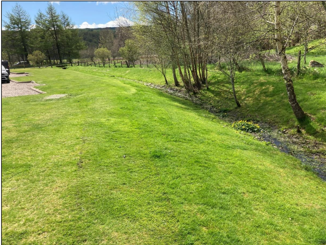
Example of a channel dug to convey hillside drainage around a car park, where naturally it would have spread
