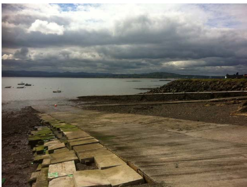
Figure 6 East Slipway showing precast block protection to east face (Chainage 280m)
