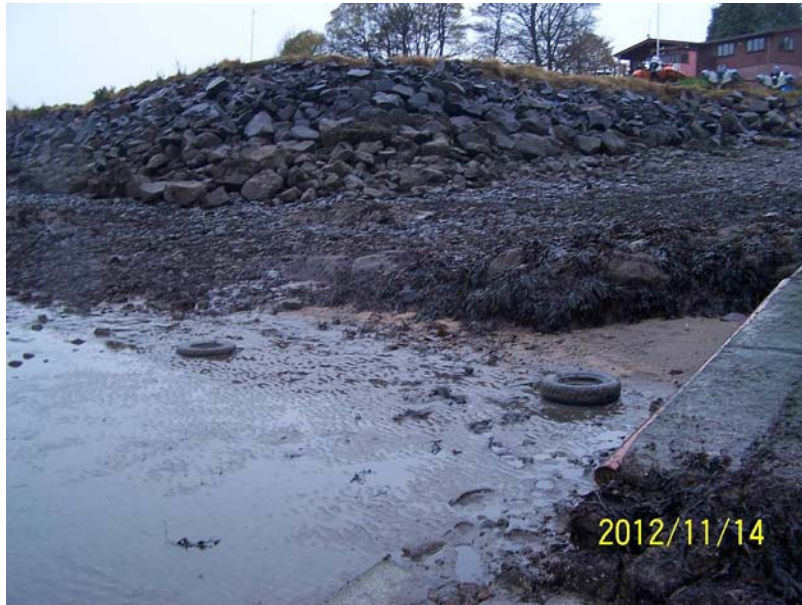
Figure 12 Coarse Sand Beach formed updrift of Jetty off Promontory 1 (Chainage 170m)
