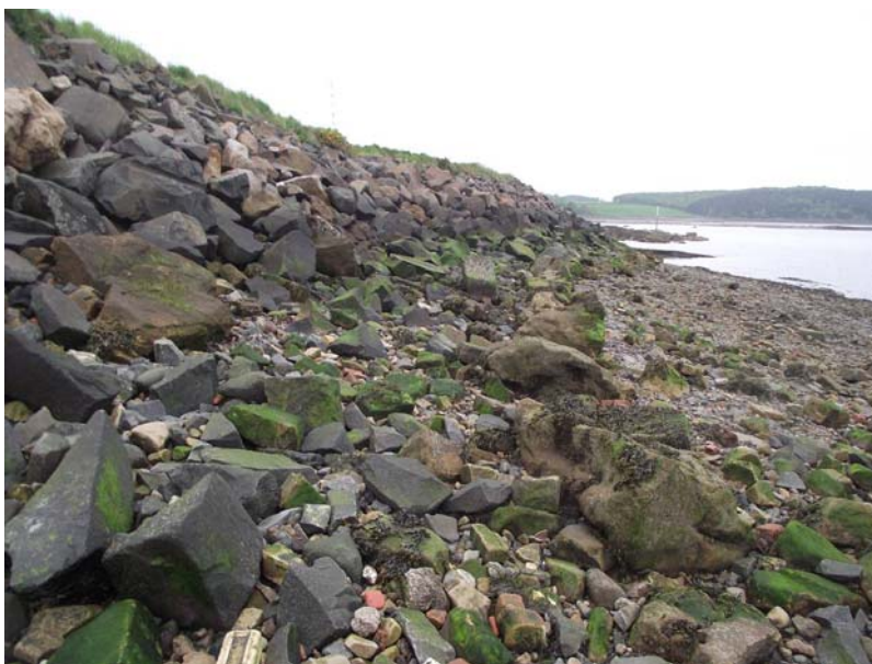
Figure 3 Armour stone to Promontory 1 (Chainage 70-140m)
