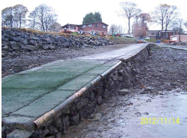
Figure 13 Groyne Effect of Jetty on beach levels
