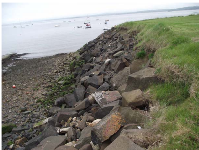
Figure 4 NE Face of Promontory 1 (Chainage 60-80m)
