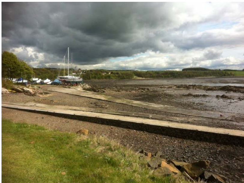
Figure 7 Showing Slipways and Promontory 2 (Chainage 300m) from Promontory 1 (Chainage 170m)
