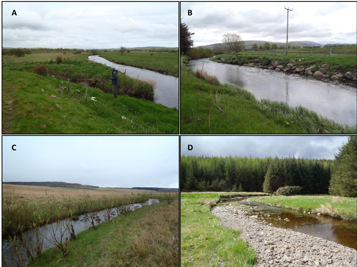
Figure C1 Nith upstream of New Cumnock – A: embanked channel near New Cumnock; B: bank protection in downstream part of water body; C: realigned reach through mining area; D: active upstream section with forestry.
