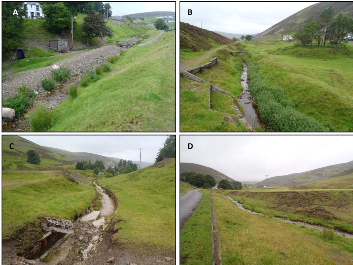
Figure C3 Wanlock Water – A: recently modified embankment; B: upper realigned section; C: dry, open culvert channel; D: lower realigned section through mine spoil.
