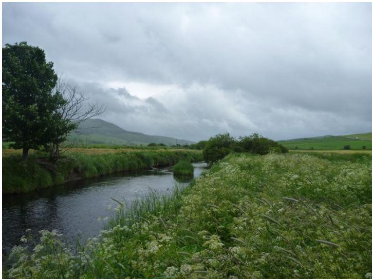
Figure H.2: River Nith within the New Cumnock model domain. Embankment on the right bank of the River Nith. Floodplain on both sides of the Nith.
