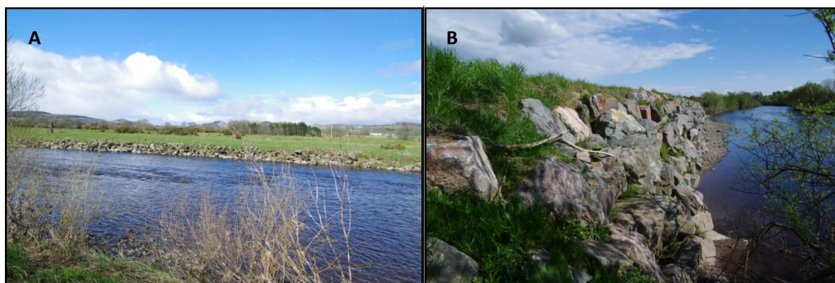
Figure 2.7 Examples of hard bank protection impacting on geomorphic process on the Nith main stem: A: near Thornhill; B: near Dumfries
