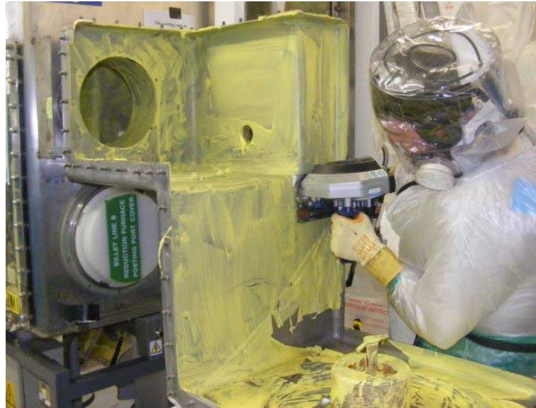
Figure 11: Use of Decontamination Agents and Strippable Coatings to Protect Workers during Decommissioning
