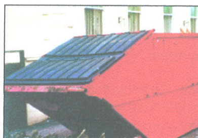
Use a lockable skip for asbestos cement sheet
