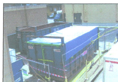
It is not good enough to throw sheeting over a standard skip
