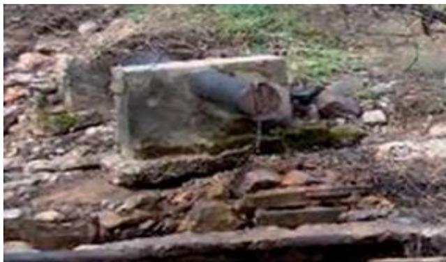
Figure 3 shows where the outfall structure extending into the channel has caused erosion (scour) of the bank, increasing sediment supply downstream and leading to damage of the structure itself
