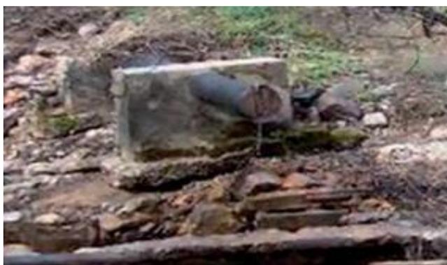
Figure 3 shows where the outfall structure extending into the channel has caused erosion (scour) of the bank, increasing sediment supply downstream and leading to damage of the structure itself
