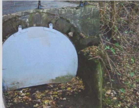
Figure 15 photograph Bank side outfall with mitred headwall
