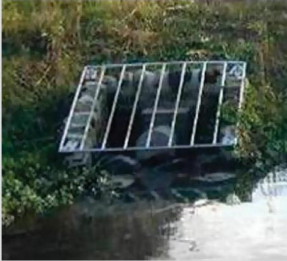
*Figure 34 screen angled at 45° to prevent debris, such as falling branches from blocking the outfall and to prevent vandalism.*
