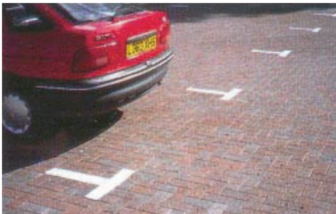
Porous paving can significantly reduce surface water run-off. © SEPA Natures Way
