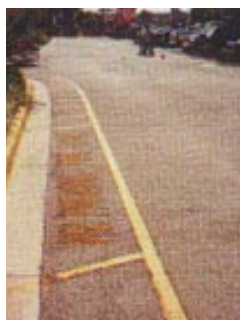
A 'porous' road surface helps to reduce run-off and pollution. © SEPA
