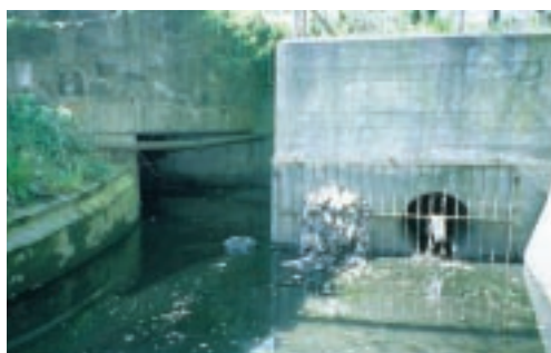
Watercourse or sewer? - or both? A typical urban stream with culverting and associated cross connection problems. Edinburgh © SEPA
