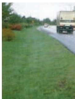
This swale will help prevent oil and heavy metals from the road from entering the river system. © SEPA
