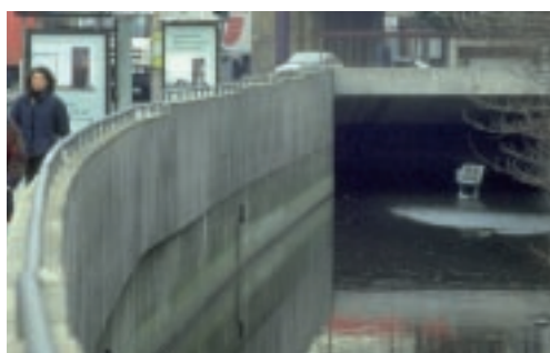
Many watercourses have been modified with one objective in mind - the unimpeded movement of water. They offer little for people or wildlife. Some have been lined with concrete to cope with the increased storm flows caused by urbanisation. © RPH
