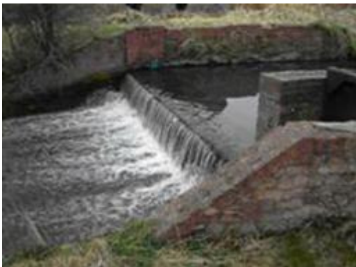
Figure 5 Artificial Control: Weir
