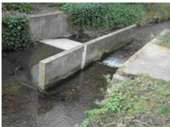
Figure 15 Compound Crump Weir
