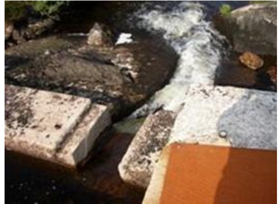
Figure 14 Broad Crested Weir With No Low Flow Structure
