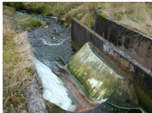
Figure 6 Artificial Control: Flume
