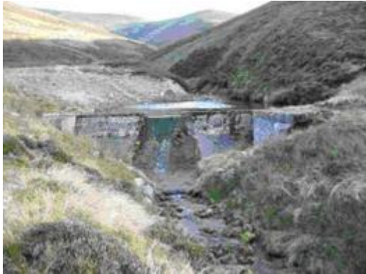
Figure 14 Broad Crested Weir With No Low Flow Structure
