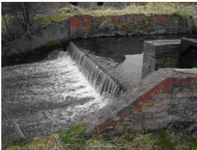
Figure 14 Broad Crested Weir With No Low Flow Structure
