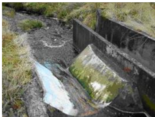
Figure 16 Trapezoidal Flume
