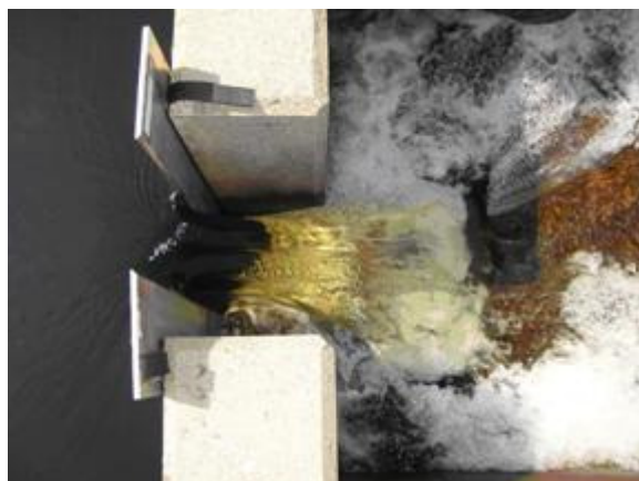
Figure 10 Rectangular Thin Plate Weir
