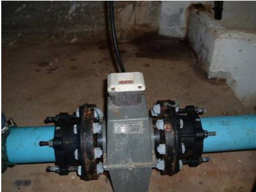
Figure 20 Electromagnetic Flow Meter
