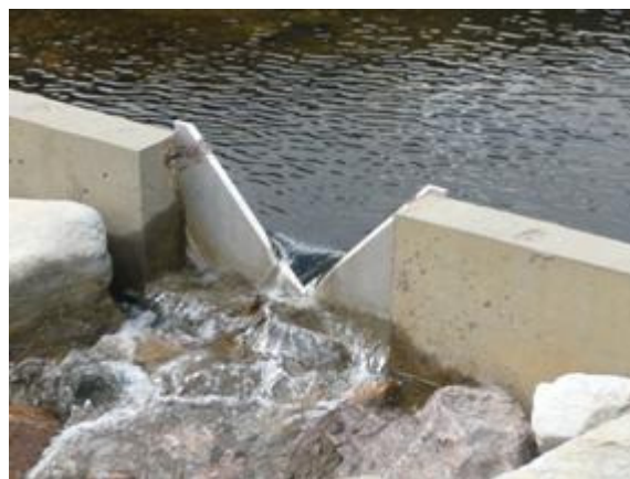
Figure 11 V-notch Thin Plate Weir
