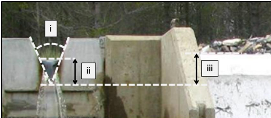
Figure 16. Mitigation Structure (V-notch)
