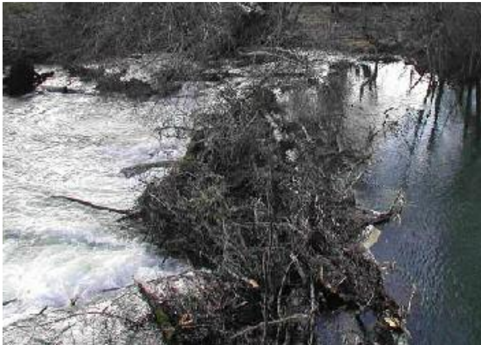
Figure 32. Same site on Rickreall Creek during moderate flow in winter 2004, showing accumulation of flotsam on the structure and the natural appearance of a complex logjam.
