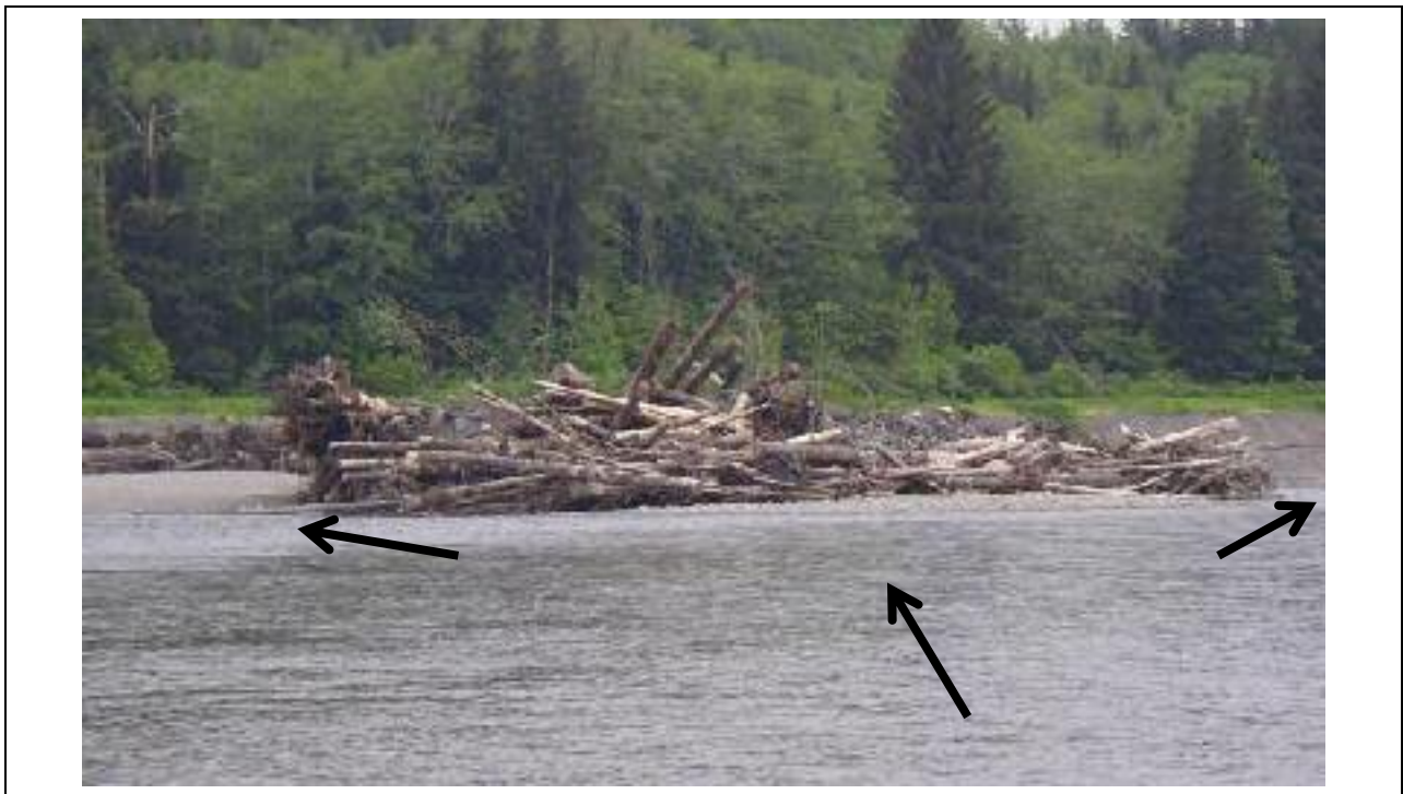
Figure 18b. Example of bar apex ELJ constructed in September 2004 in the Hoh River, Jefferson County, Washington, showing conditions in March 2005 after two peak flows of approximately 850 centimeters.
