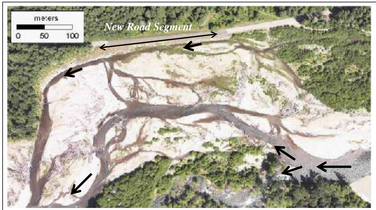
Figure 34. Site B on Cispus River in 1999 before ELJ construction where 150-meter road segment was washed out in 1996.
