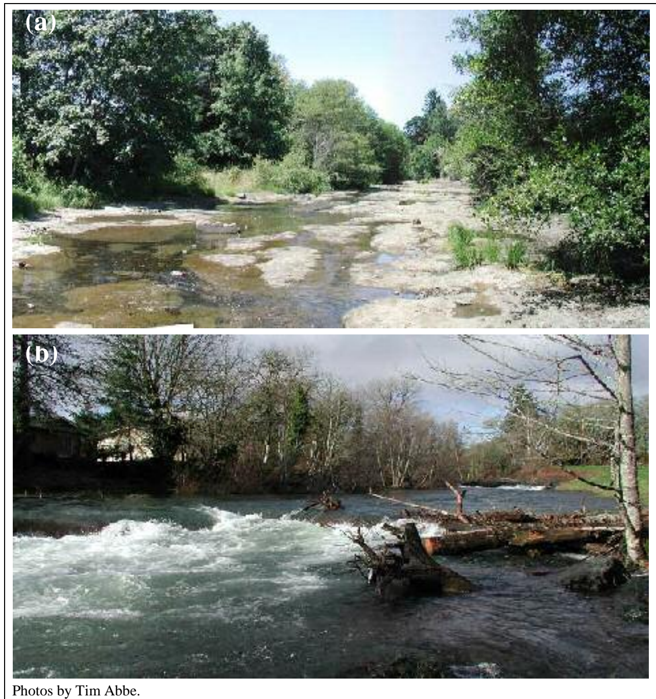
Figure 33. Conversion of incised bedrock channel to step-pool and pool-riffle channel using ELJ grade control structures in Rickreall Creek, Dallas, Oregon: (a) conditions during summer low flow in 2002, before project construction and (b) conditions during winter peak flow in 2004, after project construction (flow is from upper right to lower left).
