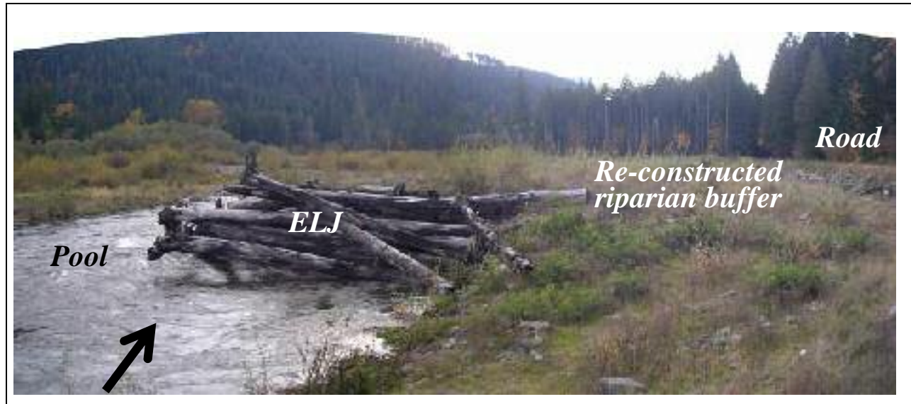
Figure 36. One of four flow deflection ELJs in Cispus River constructed to increase pool frequency and cover, improve riparian conditions, and protect the road, 5 years after construction (November 2004).
