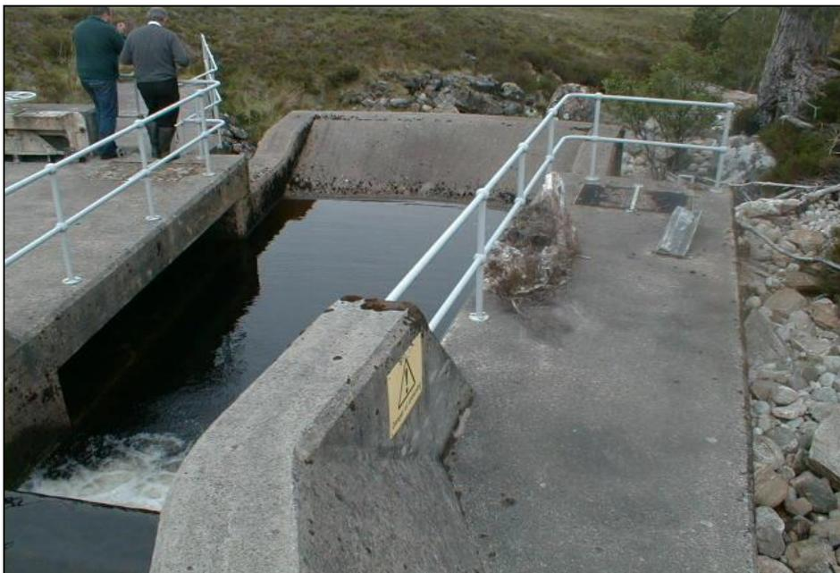
**Picture 1:** Scoop intake showing 'scoop' shaped central channel with side intakes. In high flow conditions the water continues over the crest of the intake and effectively scours the intake on every spill (photograph courtesy of Scottish & Southern Energy).
