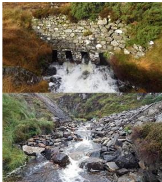
Figure 2: September 2016 – Culvert removed and channel remedial work progressing.
