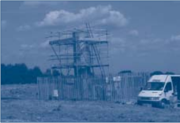
Figure 5.5 Two-stage sampling platform for monitoring emissions from a landfill gas flare
