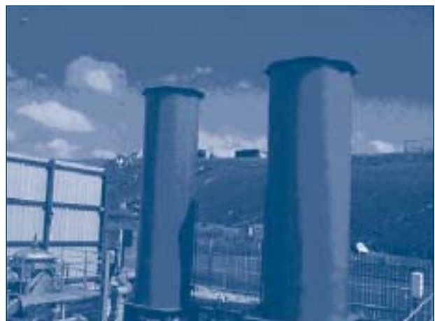
Figure 3.2 | An example enclosed flare
