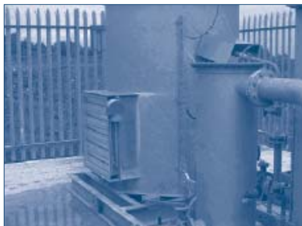
Figure 3.3 Air control louvres employed on an enclosed flare
