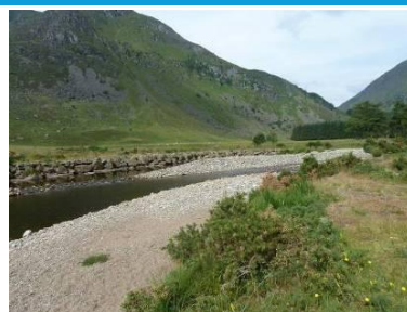
Boulder bank protection
