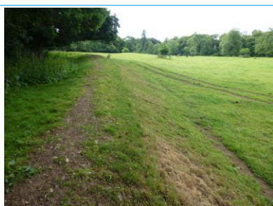
Disconnected floodplain via embankment
