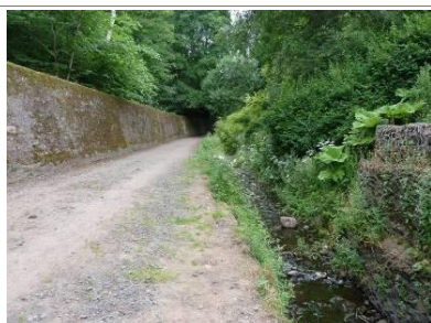
Artificially straightened and lined channel
