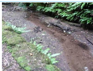
Build up of silt and fine sediment
