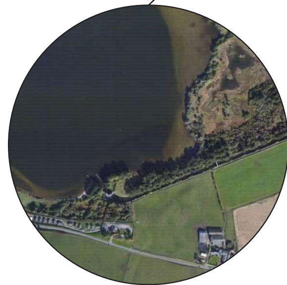
Site: Loch Leven sluice
