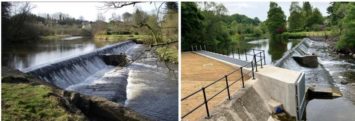
Figure 1 – Mid Calder Weir before (left) and after fish pass installation.
