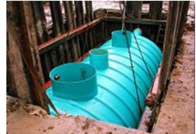
Example of a full retention separator during installation.
