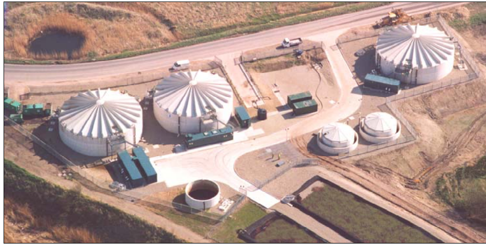
Plate 2.16: Large tank-based SBR System: Arpley Landfill, Warrington, 450 m 3 /d (COD 10,000 mg/l, ammoniacal-N 2500 mg/l), 2001- (see Robinson and Last, 2003)
