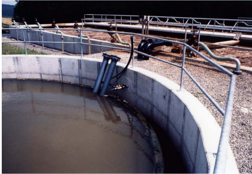
Plate 2.11: Typical application of the activated sludge process to leachate treatment, showing sludge settlement in the foreground, and aeration reactor in the background, Germany, 1990
