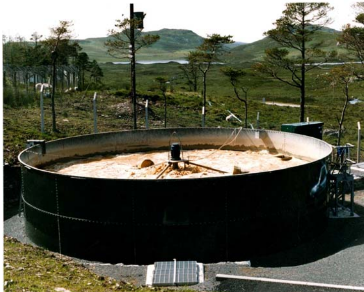
Plate 2.17: Smaller tank-based SBR treating leachate at Gairloch Landfill, Ross and Cromarty (30 m 3 /d, 1993-)
