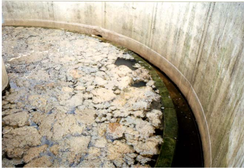
Plate 2.12: Rising sludge as a consequence of denitrification within the settlement phase of an activated sludge system treating leachate, Germany, 1990
