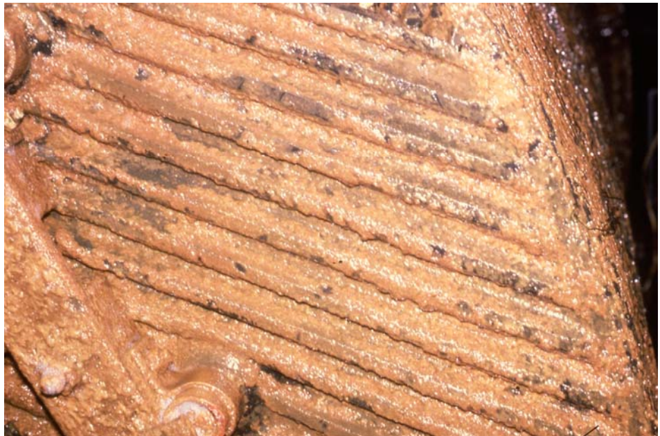
Plate 2.19: Growth of biofilm on RBC media at Pitsea RBC Plant
