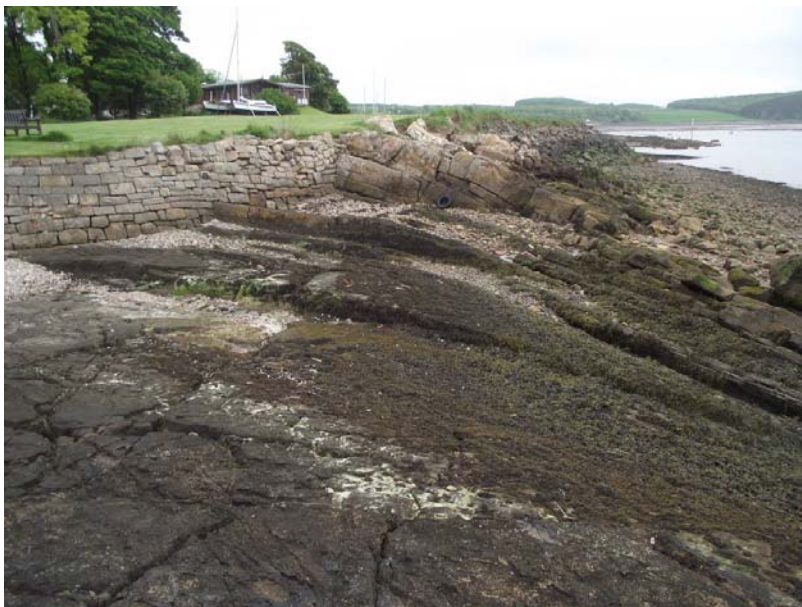
Figure 2 Rock foreshore & Raised Beach (chainage 40 to 50m)
