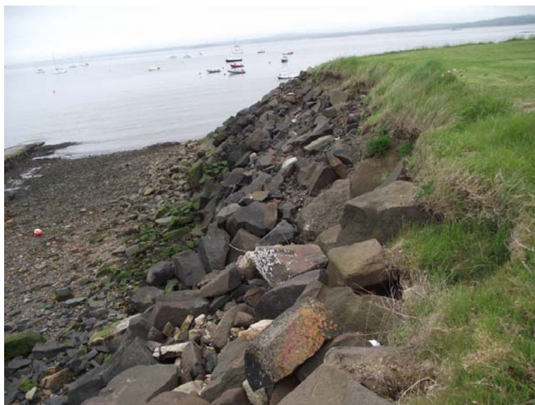
Figure 4 NE Face of Promontory 1 (Chainage 60-80m)
