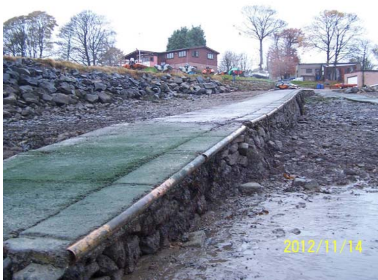
Figure 13 Groyne Effect of Jetty on beach levels
