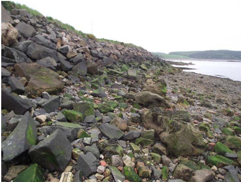
Figure 3 Armour stone to Promontory 1 (Chainage 70-140m)
