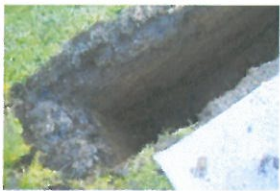
TP2-4-021 Open Excavation (8)
