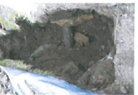
P2-3-018 Open Excavation (4)
