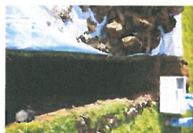
TP1-1-008 Open Excavation (1)
