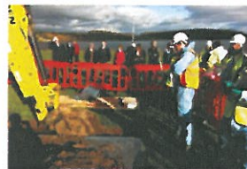
TP1-1-008 Excavation and Forum Observation
