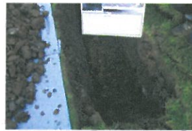
P2-1-013 Open Excavation (1)
