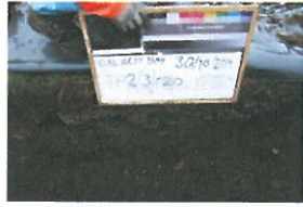
TP2-3-020 Open Excavation
