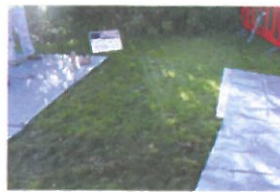
TP2-4-021 Before Excavation (4)
