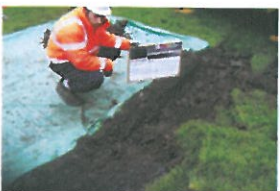
TP2-1-012B Open Excavation (7)
