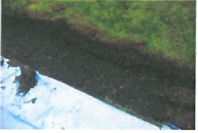
TP2-1-009 Open Excavation (2)
