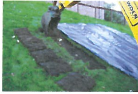
P2-2-015 Open Excavation below 1m
