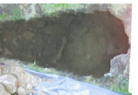
P2-3-019 Open Excavation (1)
