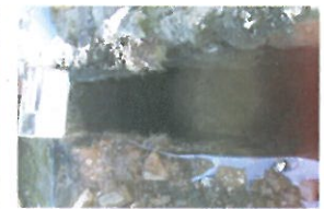
TP1-1-007 Open Excavation (15)
