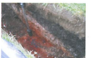
P2-2-015 Open Excavation (12)
