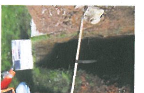
P2-2-015 Open Excavation (17)
