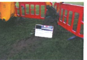
TP2-1-009 Before Excavation (2)
