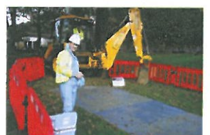
TP2-1-011 Before Excavation (1)
