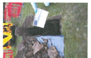
P2-3-018 Open Excavation (3)
