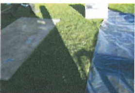
P2-3-019 Before Excavation (4)
