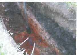
P2-2-015 Open Excavation (13)
