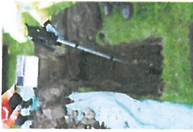
TP2-1-012 Open Excavation (2)
