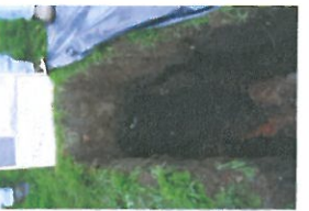
P2-2-015 Open Excavation (5)
