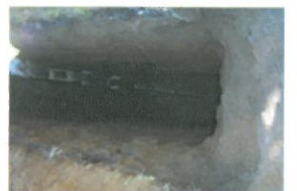
TP2-4-021 Open Excavation (11)
