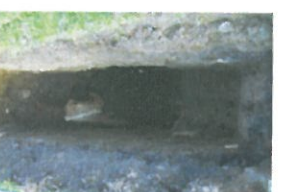
TP2-1-013 Open Excavation (6)
