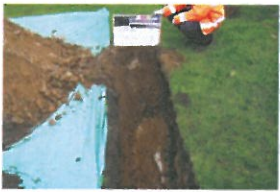
TP2-1-014 Open Excavation
