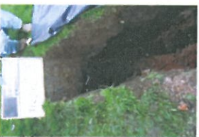
P2-2-015 Open Excavation (7)
