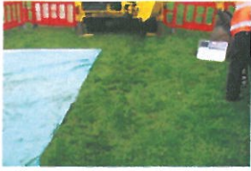
TP2-1-012 Before Excavation (2)
