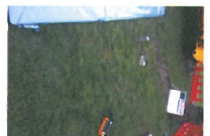
TP2-1-009 Before Excavation (2)
