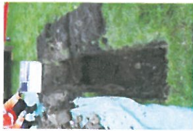
TP2-1-012 Open Excavation
