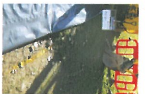
TP1-1-007 Before Excavation
