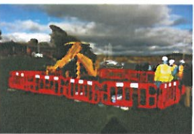
TP1-1-008 Excavation Area (10)
