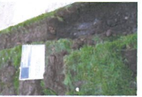
P2-2-016 Open Excavation (4)
