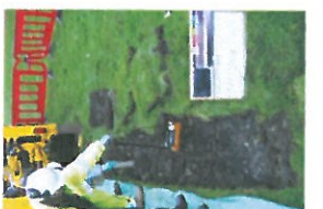
TP2-1-012B Open Excavation (8)
