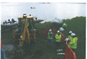
P2-2-015 Open Excavation (11)
