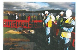
TP1-1-008 Excavation and Forum Observation
