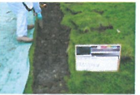
TP2-1-012B Open Excavation (9)
