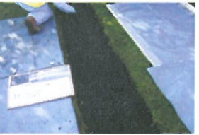
TP2-4-021 Open Excavation (5)
