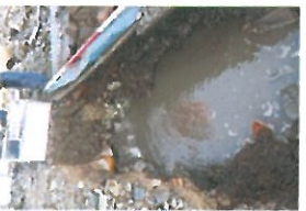
TP7-2-081 Open Excavation (5)
