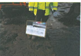
TP7-2-078 Before Excavation
