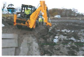
TP7-2-102 Restored Surface 4
