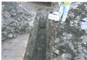
TP7-2-102 Open Excavation 2
