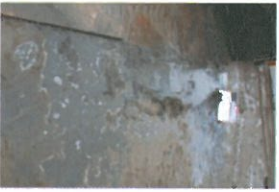
P-NH-094 Restored Surface (3)
