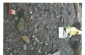
TP7-2-081 Before Excavation
