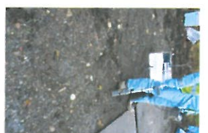
P7-2-070 Before Excavation (6)
