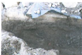
P7-2-074 Open Excavation (6)
