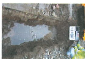
TP7-2-101 Open Excavation
