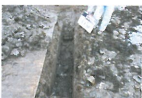
TP7-2-102 Open Excavation
