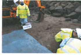
TP7-2-100 Before Excavation
