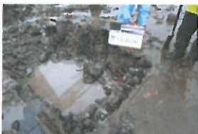
TP7-2-098 Open Excavation 2
