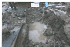
TP7-2-098 Open Excavation
