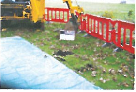
TPNH096 Before Excavation (1)
