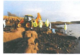
TP7-2-099 View of Excavation Area
