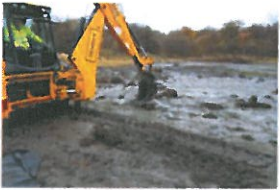
P7-2-067 Before Excavation & Construction
