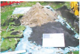
TPNH096 Open Excavation (8)
