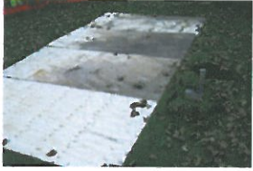
TPNH096 Before Excavation (1)
