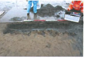
P-NH-094 Open Excavation (8)
