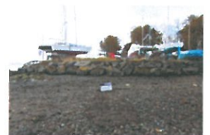
TP7-2-080 Restored Surface and Compaction
