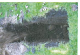
TPNH095 Open Excavation 17
