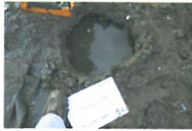
P-NH-093 Open Excavation (3)
