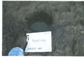
P-NH-092 Open Excavation (3)
