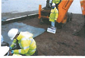
TP7-2-100 Before Excavation
