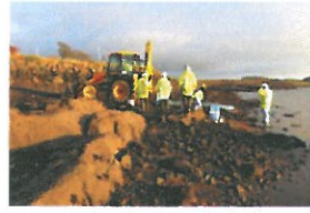
TP7-2-099 View of Excavation Area
