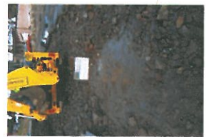
P7-2-083 Restored Surface (7)
