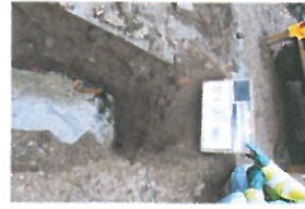
TP7-2-100 Open Excavation 2
