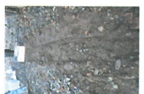
TP7-2-101 Restored Surface
