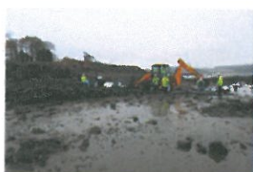
TP7-2-098 View of Excavation Area
