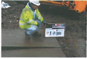
TP7-2-102 Restored Surface 2
