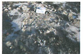
TP8-1-105 Restored Surface
