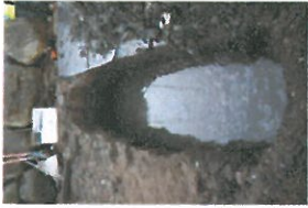
TP7-2-076 Open Excavation (2)
