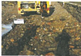
P7-2-084 Before Excavation (2)
