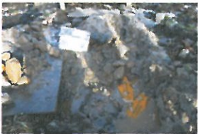
TP8-1-105 Open Excavation
