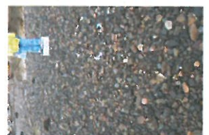
TP7-2-101 Before Excavation
