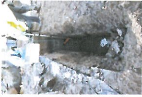
TP7-2-079 Open Excavation (1)
