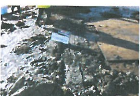
TP7-2-078 Restored Surface (1)
