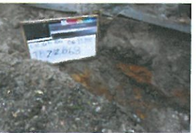
P7-2-068 Open Excavation (2)
