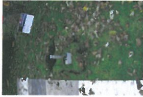
TPNH096 Before Excavation (1)
