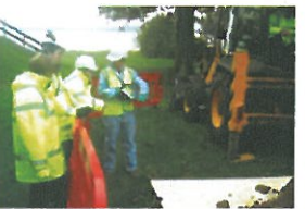
TPNH095 Excavation Setting 8
