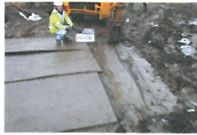
TP7-2-102 Restored Surface
