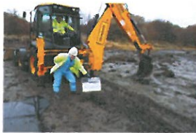
P7-2-067 Before Excavation (6)
