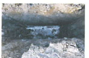
TP7-2-078 Open Excavation (6)
