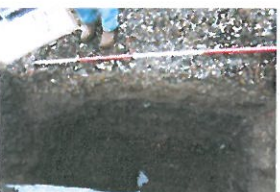
TP7-2-082 Open Excavation (8)
