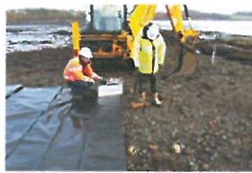
TP7-2-080 Before Excavation
