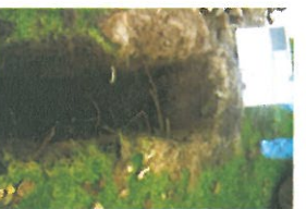
TPNH095 Open Excavation 12
