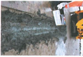
P-NH-094 Open Excavation (3)
