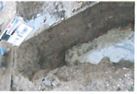
TP7-2-100 Open Excavation 4
