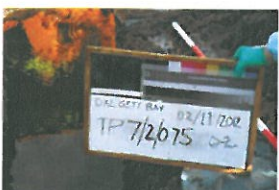
P7-2-075 Open Excavation (4)
