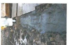
TP7-2-099 Restored Surface
