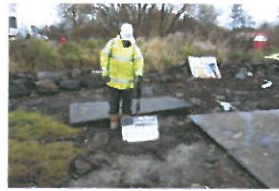
P7-2-066 Before Excavation (6)
