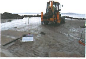
TP-NH-094 Before Excavation
