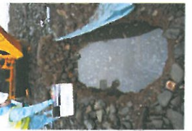
P7-2-085 Open Excavation (3)
