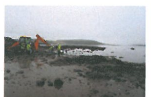
TP7-2-098 View of Excavation Area
