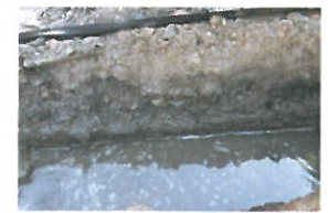
TP7-2-079 Open Excavation (6)
