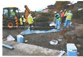
P7-2-082 Spoil and Excavation Area
