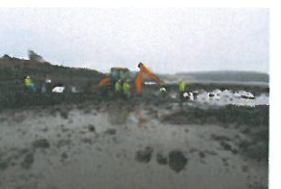
TP7-2-098 View of Excavation Area
