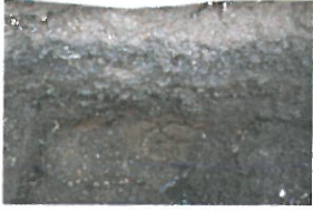
P7-2-082 Open Excavation (1)
