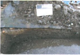
TP7-2-076 Open Excavation and Spoil
