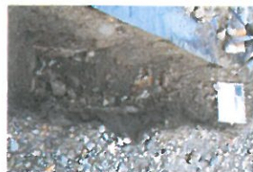
TP7-2-080 Open Excavation (10)
