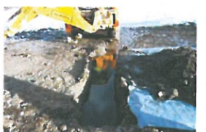
P7-2-075 Open Excavation (5)
