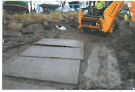
TP7-2-102 Restored Surface 3
