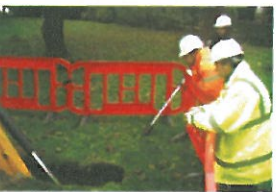
TPNH095 Open Excavation 7
