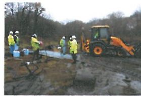
TP7-2-097 Before Excavation View
