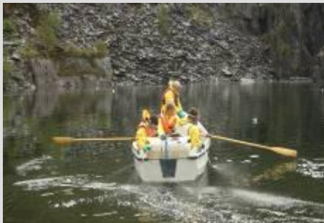
Pyblast being applied to the pond using boat-mounted sprayers
