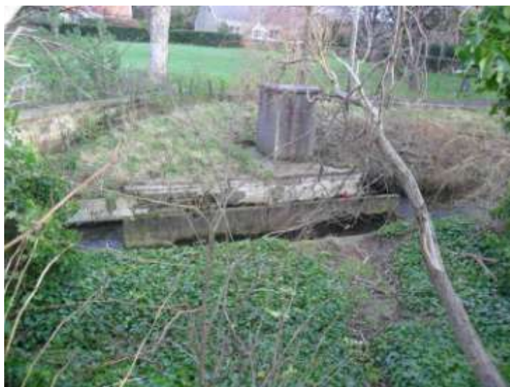
Figure 1-21: SEPA gauge at Liberton Upstream of Cameron Toll Shopping Centre
