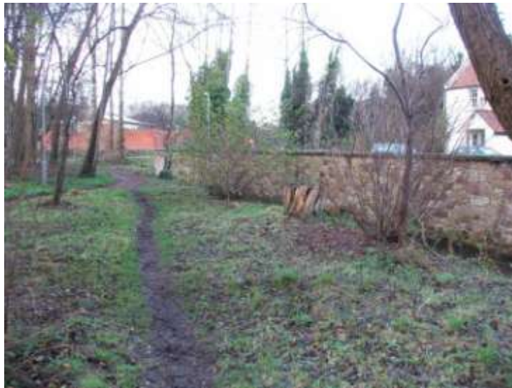
Figure 1-20: Small wet woodland near Cameron Toll showing floodwall and low levee
