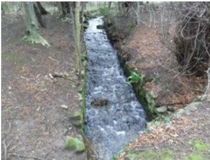
Figure 1-5: Lined reach of the upper Braid Burn
