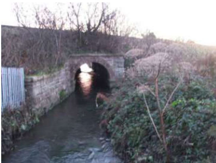
Figure 1-26: Railway culvert at Peffermill with giant hogweed on the left bank, where the drain joins the main channel
