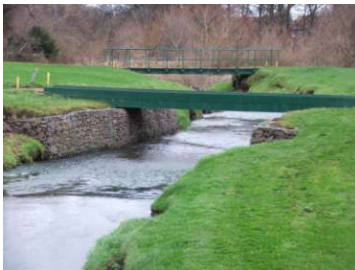
Figure 1-34: Gabion baskets lining the Braid Burn in Duddingston Park
