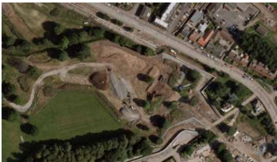
Figure 1-22: Floodwalls and wetland being constructed in Inch Park (Google Maps 2012)
