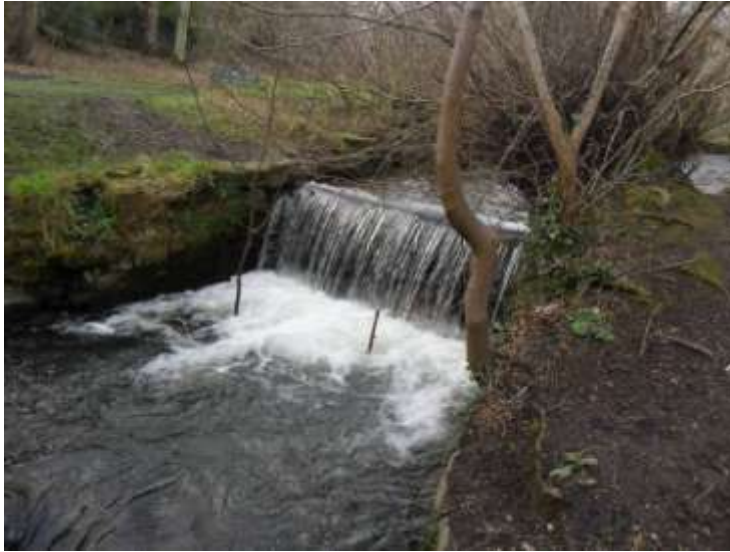
Figure 1-16: Small weirs along the Braid Burn through the Hermitage of Braid
