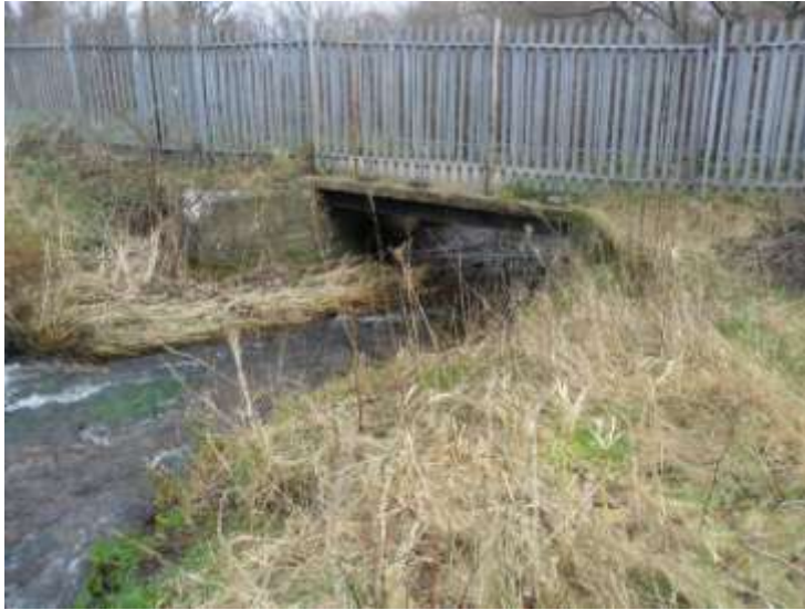
Figure 1-10: Concrete footbridge over the Braid Burn
