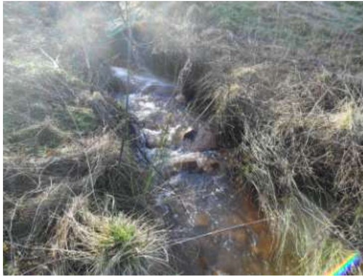
Figure 1-13: Masonry rapids in the channel after Inchcross Road.
