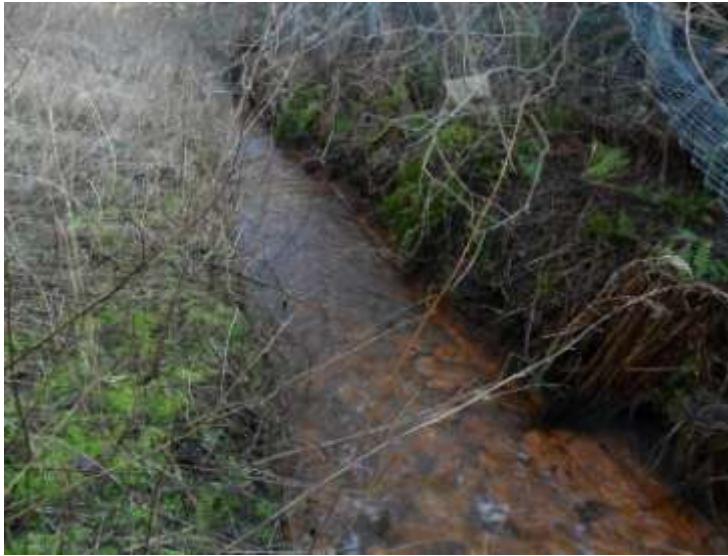
Figure 1-11: Brick lined channel through Standhill.
