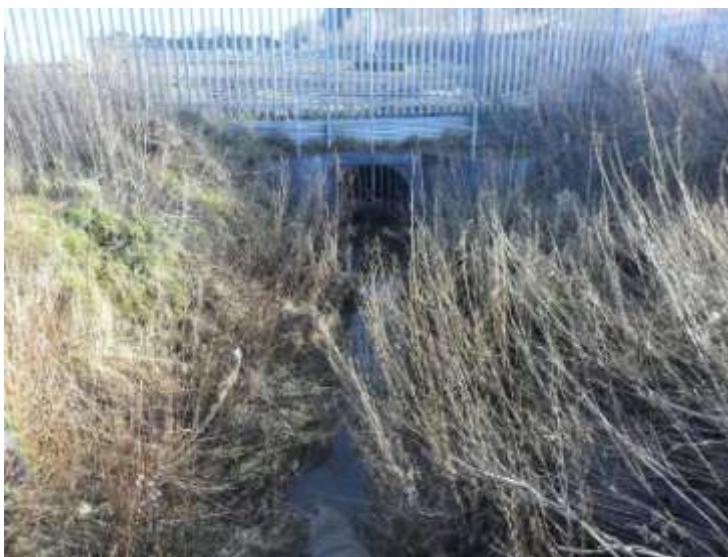
Figure 1-10: The culvert under Standhill Depot
