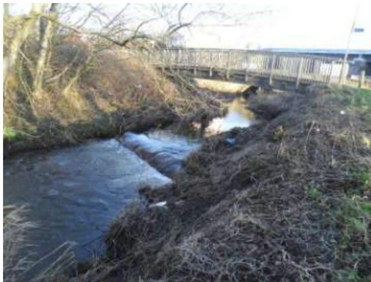
Figure 1-18: Low flow control on Bog Burn
