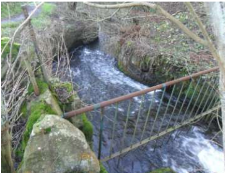
Figure 1-9: Weir structure controlling flow into Coul Reservoir
