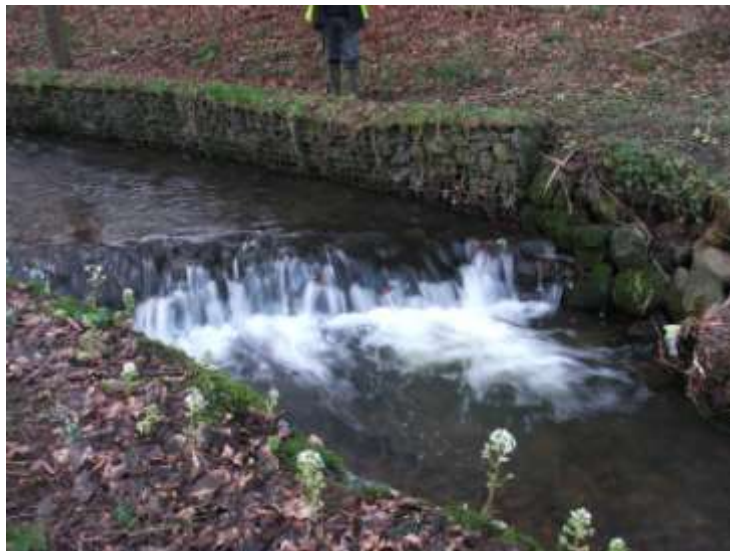
Figure 1-29: Gabion baskets and cobble weir hindering fish passage and the development of a riparian margin
