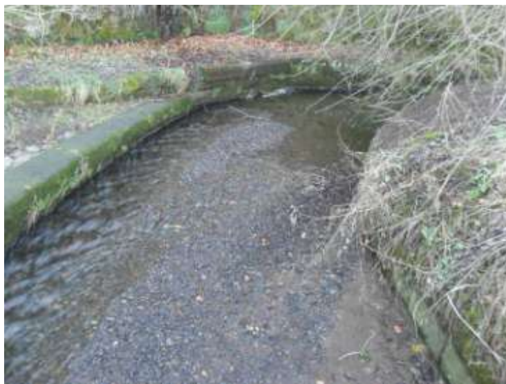
Figure 1-10: Mixed sediment deposition upstream of the weir controlling flow into Coul Reservoir
