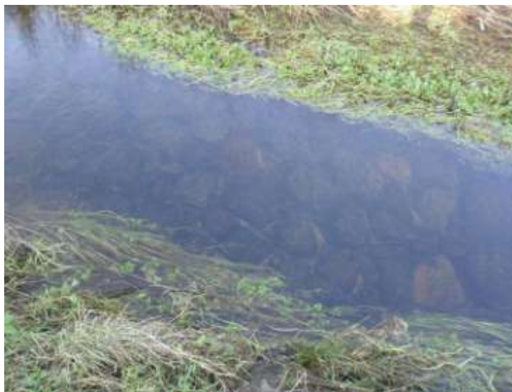
Figure 1-6: Detail of the cobble lined raceway
