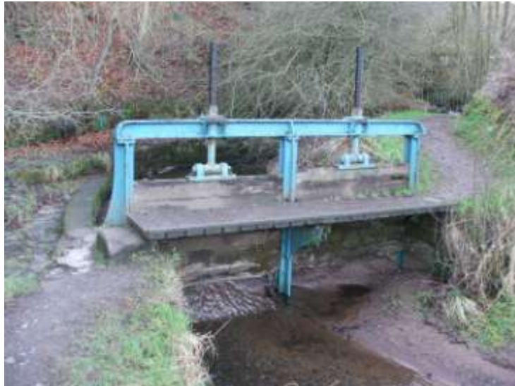
Figure 1-5: Victorian cast iron sluice gate used to direct water out of the natural course of the burn and into a raceway
