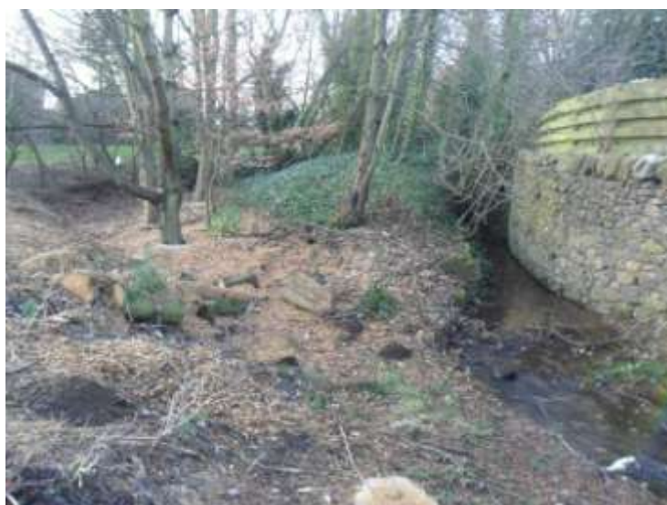
Figure 1-22: Split channel with flow confined to the artificial section
