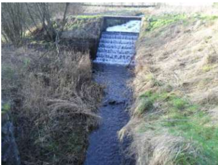
Figure 1-13: Walled reach at the exit weir from the raceway and gabion lined reservoir outflow channel
