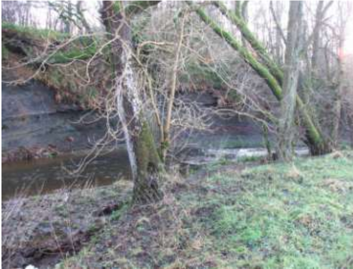
Figure 1-15: Bedrock Exposed by Erosion Just Upstream of Black Devon Bridge
