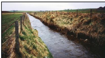
Figure 1.8 Fedderate Water, tributary of the South Ugie Water, Aberdeenshire. Photo on left ca. 1990 immediately following maintenance dredging. Centre photograph was taken in the summer following the first photograph showing the limited extent to which vegetation recovered in six months. Right photo, recent photo from Google Street View shows how vegetation has encroached on the channel. Again, this channel is clearly stable and does not erode, except when freshly dredged.
