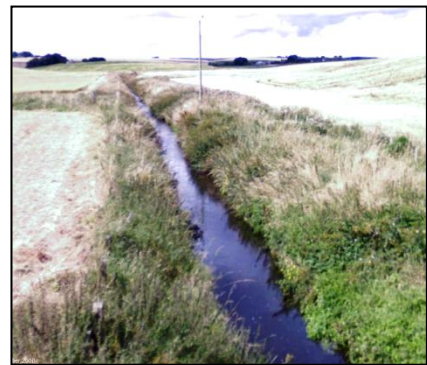
Figure 1.8 Fedderate Water, tributary of the South Ugie Water, Aberdeenshire. Photo on left ca. 1990 immediately following maintenance dredging. Centre photograph was taken in the summer following the first photograph showing the limited extent to which vegetation recovered in six months. Right photo, recent photo from Google Street View shows how vegetation has encroached on the channel. Again, this channel is clearly stable and does not erode, except when freshly dredged.
