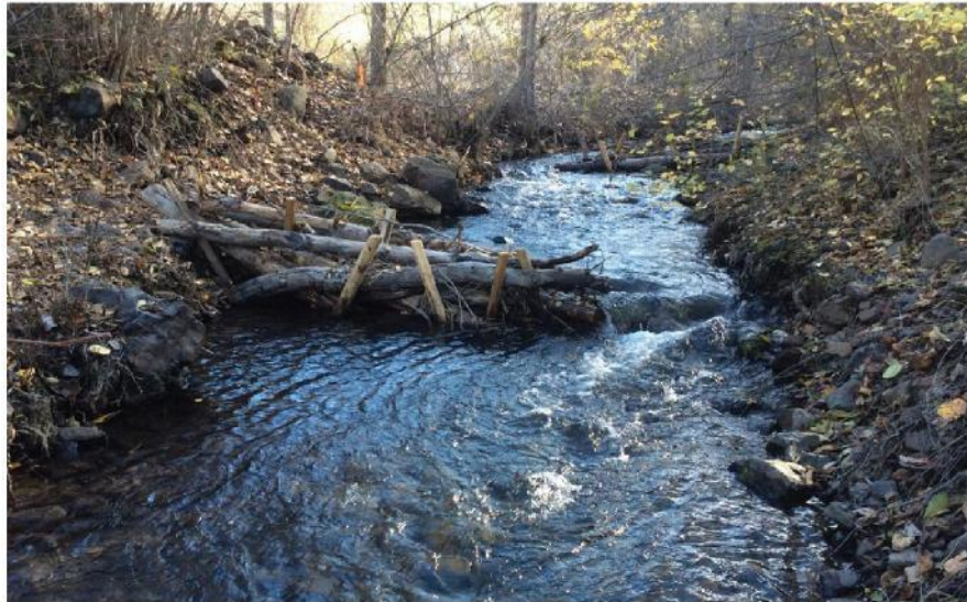
Figure 40: Photograph of bank-attached ELJs, designed to enhance channel diversity. Sourced from Wheaton et al. 2019.
