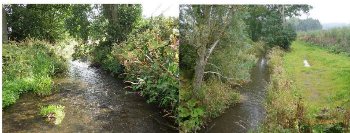
Figure 65: The photograph on the left shows the general state of the channel prior to restoration and the photograph on the right shows the 2-stage channel which was installed with the new section of floodplain on the right bank (looking downstream). Deflectors have been installed since this photo was taken which will encourage the river to adjust within this floodplain section.
