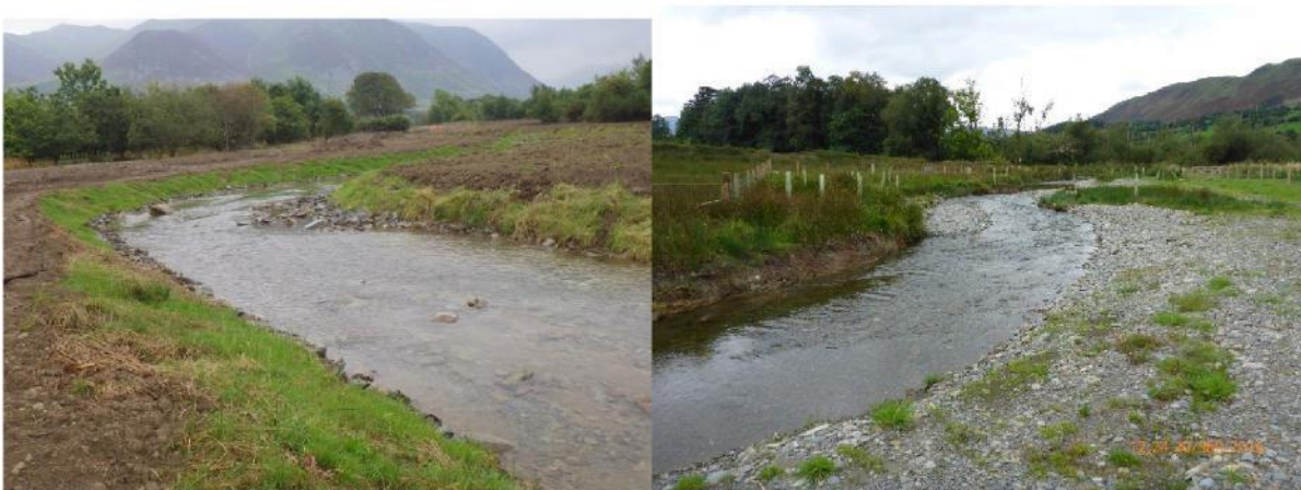
Figure 46: Examples of habitat in the remeandered Whit Beck, in Cumbria following restoration. A) shows Whit Beck 1 week after the channel was restored in August 2014 and B) shows it 2 years after it was remeandered in September 2016. This demonstrates how the channel has to actively sort its bed and rework the banks, to create the habitat appropriate for its location.
