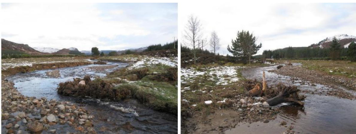
Figure 39: Examples of how wood has been used on the Aberarder restoration scheme to increase in-channel diversity and help the channel recover following remeandering. These photos were taken shortly after restoration. Photos taken November 17 by Alice Tree.
