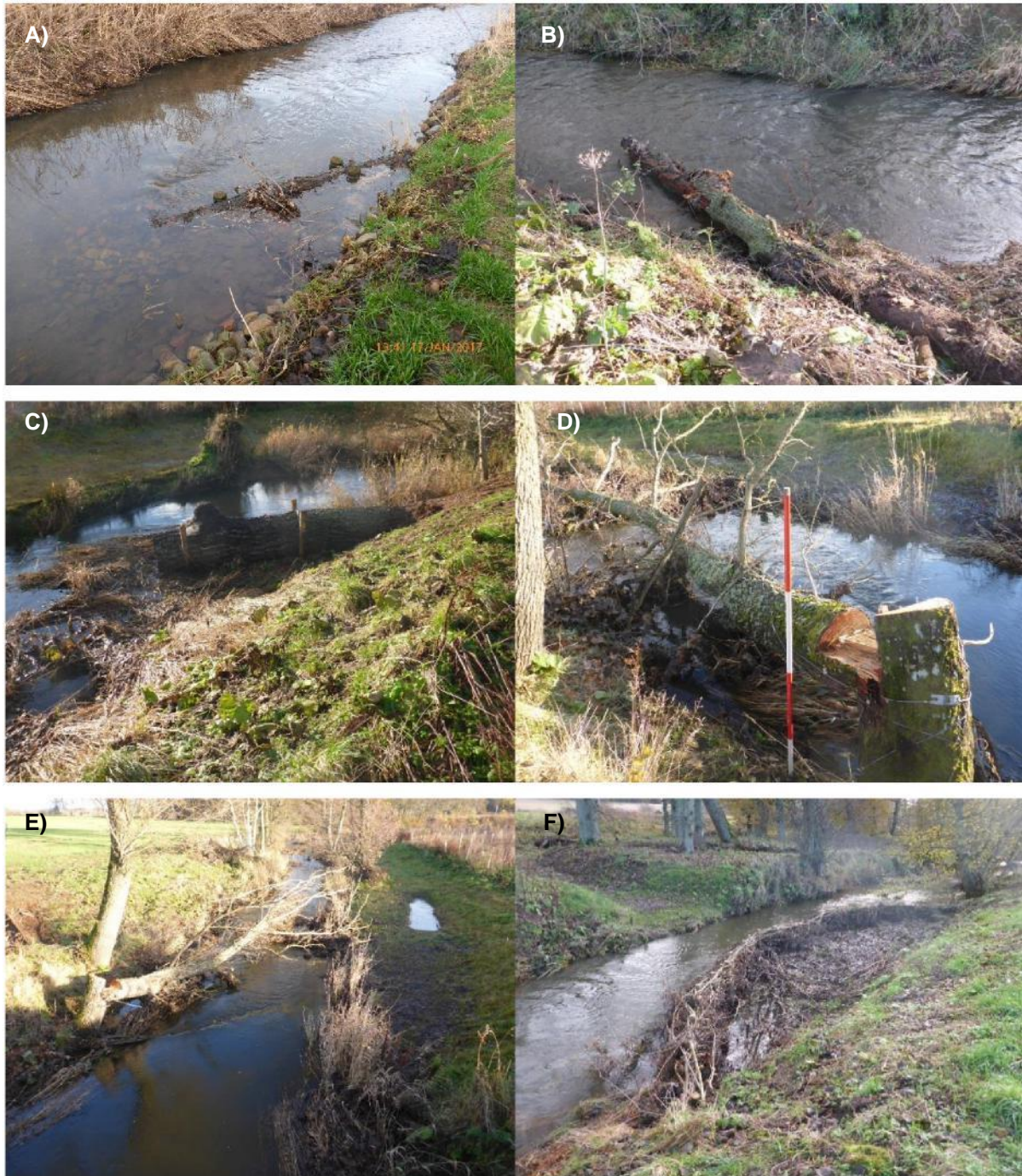
Figure 66: Examples of deflectors used in the Pow Burn scheme. A) shows the original deflectors which were installed which were seen to be undersized and not causing the erosion and creating the channel diversity necessary to upgrade morphology. B) shows a larger, rougher wood deflector, C) a log which was installed, D) and E) how live trees can be hinged into the channel and F) a willow spiling deflector designed to narrow the river.
