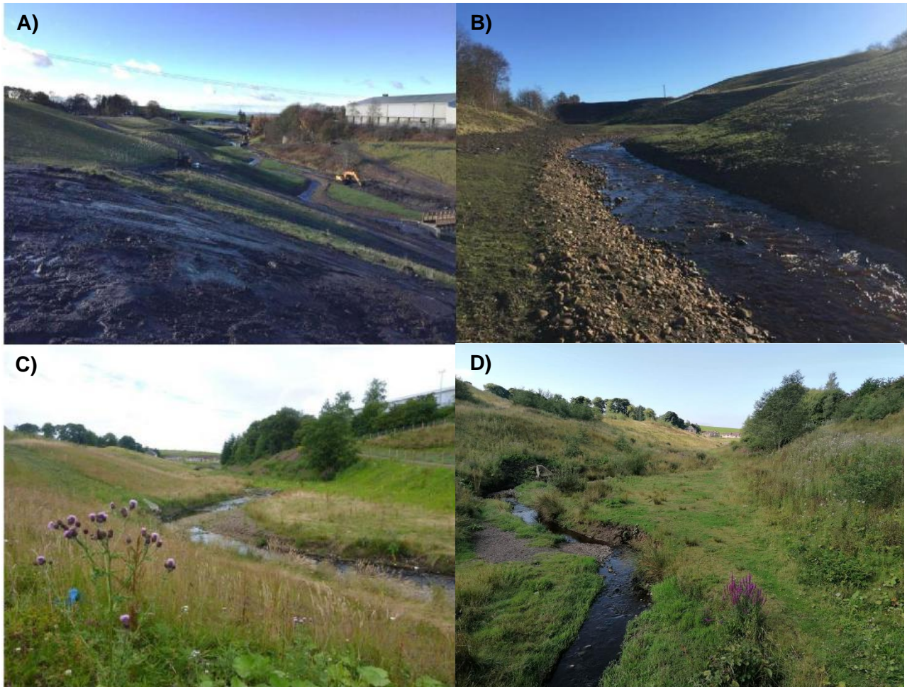
Figure 53: A) removal of the old channel after the river had been diverted into the new one, November 2016. B) Looking upstream at the newly connected restored reach in March 2016, C) looking at the restored reach in August 2017, almost 1 year following restoration and D) in 2021 5 years post restoration showing the recovery that has occurred in the form of bars, pools and riffles. Photos from Alan McCulloch and Francis Hayes.
