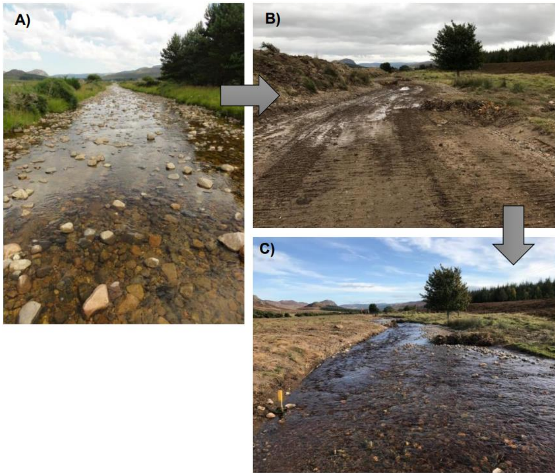
Figure 57: Photographs showing the sequence of restoration from A) pre-restoration channel taken 20 th Sept 17, B) during construction of the new channel also taken 20 th Sept 17 and C) post-restoration 9 th of October 17. This shows the very high potential for physical adjustment at the site as this adjustment was caused by a single event which was smaller than bankfull flow. Photos taken by H. Moir (cbec).
