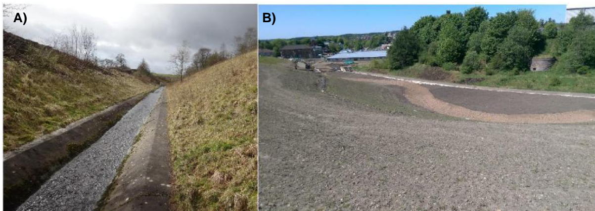
Figure 52: A) The south Calder at Stane Gardens prior to restoration showing the straight, concrete lined channel with steep valley margins. B) shows the river immediately post restoration showing how an inset valley was created and a sinuous channel within this. Photos from Alan McCulloch.
