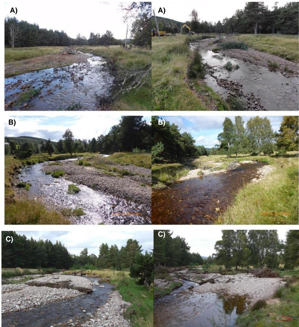
Figure 62: Photos of sections of the Allt Lorgy that have adjusted following the assisted natural recovery restoration. Note the locations of large woody material at the upstream of bars helping to increase channel sinuosity. Those photos marked A) show the river immediately after the works were completed in September 2012, B) in Sept 2016 and C) in September 2019 (supplied by Richard Williams). Thus, these all show the successive adjustment and recovery of the river.
