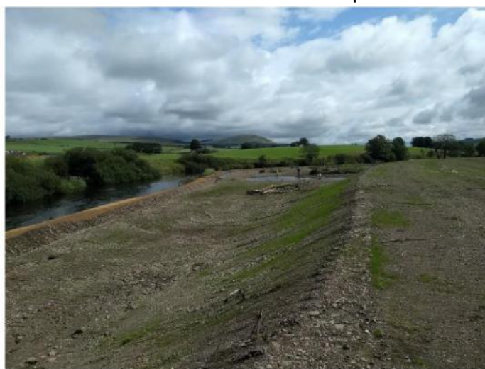
Figure 48: Photograph of the inset floodplain and set-back embankment on the River Nith taken 1 month after construction had finished in August 2019.
