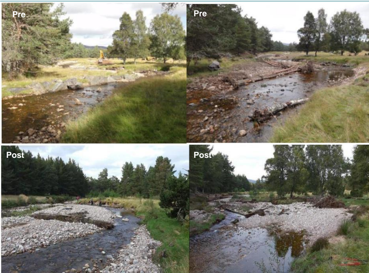
Figure G: Pre and seven years post restoration photographs of the restored section of the Allt Lorgy showing the dramatic increase in channel diversity following embankment removal and installation of wood to increase channel diversity. Pre photos supplied by H. Moir, cbec and post by Richard Williams, University of Glasgow.
