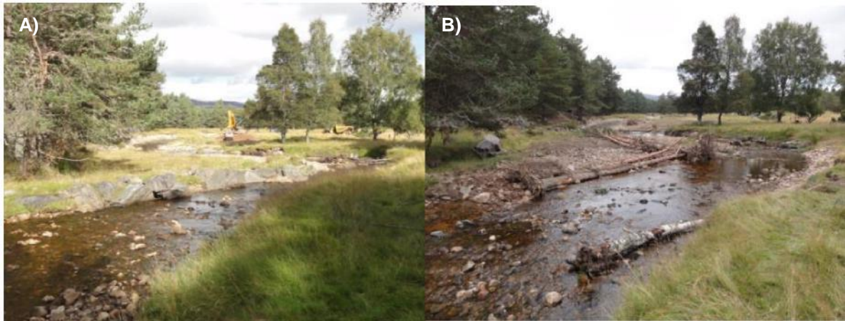
Figure 61: Photographs showing A) the boulders which lined sections of the banks which were removed and B) wood structures immediately after installation which were put in to increase channel diversity. Photos from H. Moir, cbec).
