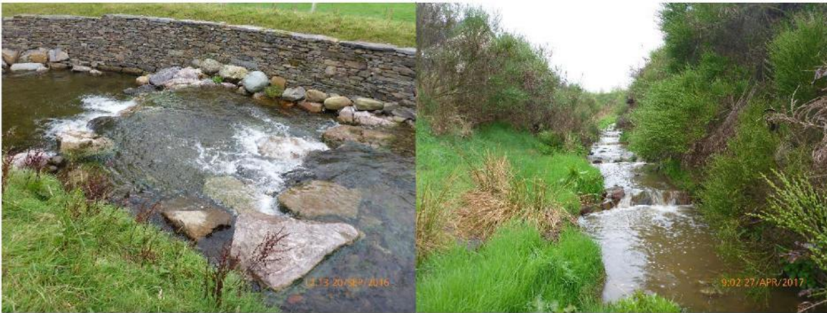
Figure 45: Examples of constructed step-pool systems that have been used in restoration schemes. A) shows steps installed in the upper tie in of Whit Beck, to hold the bed where the more constrained reach flows into the restored reach. B) more natural restored step-pool on the Mains of Dyce ~ 10 years following construction.
