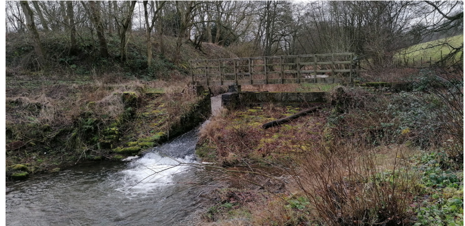
Before – Gateside Mills fish barrier in January 2022
